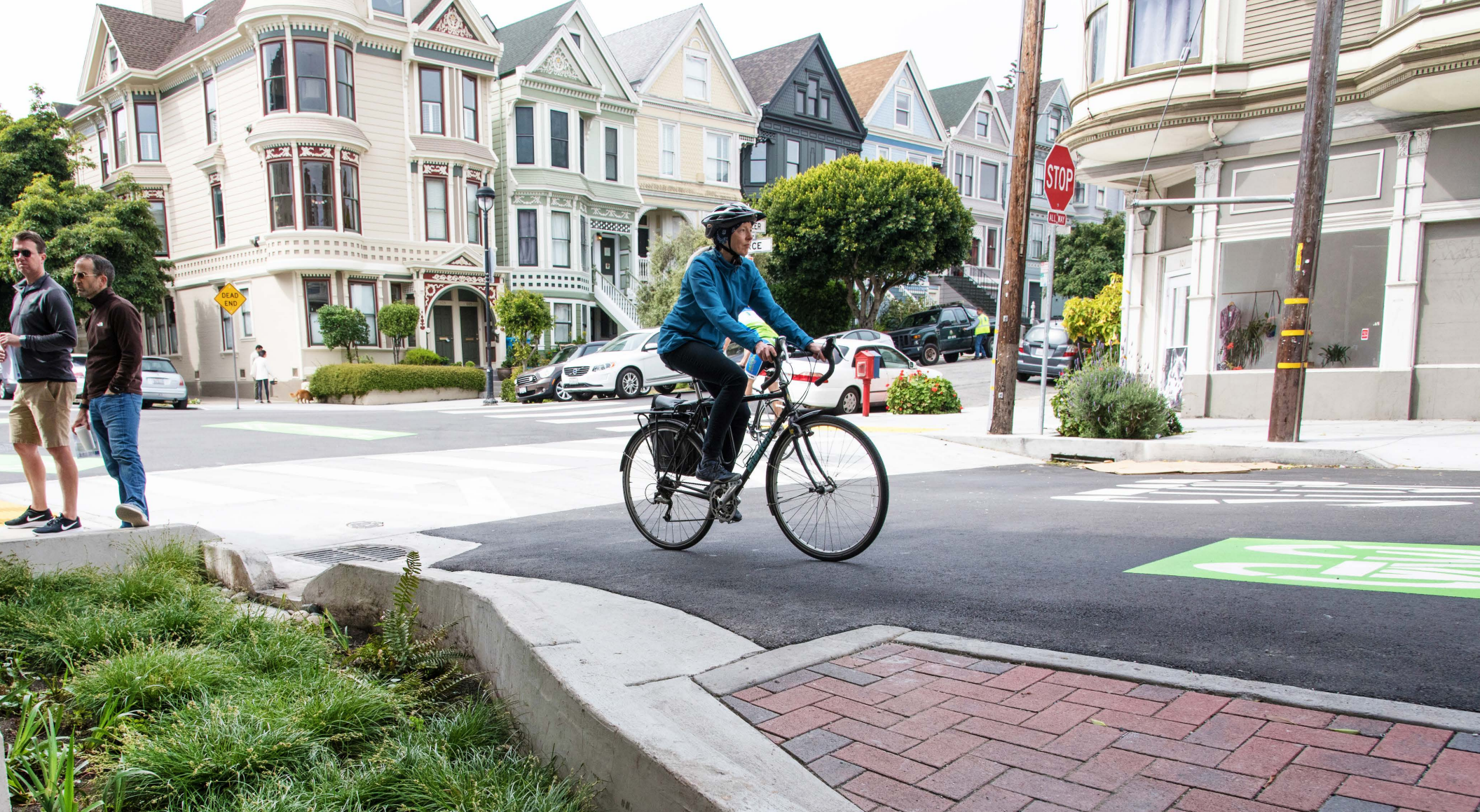
Bioretention and Permeable Pavement, Wiggle Neighborhood Green Corridor, San Francisco
