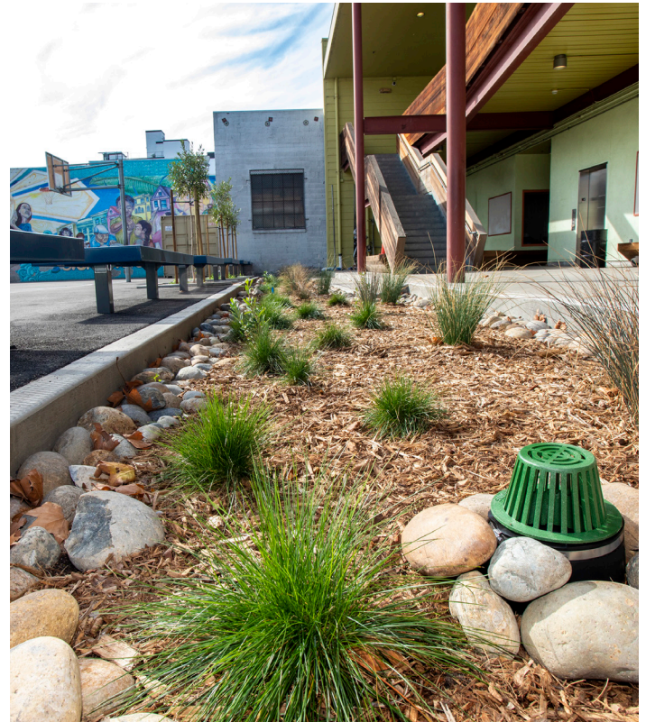
Bessie Carmichael Middle School Green Schoolyard and Green Infrastructure Grant Project: Rain garden and bioretention planters.
