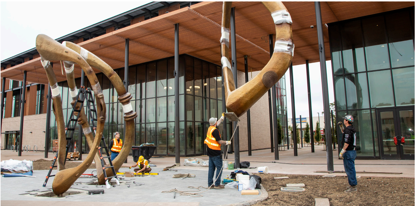
Southeast Community Center at 1550 Evans Avenue & 3rd Street: Internationally acclaimed artist Mildred Howard has been selected to create a sculpture that will be a centerpiece of the San Francisco Public Utilities Commission's (SFPUC) new Southeast Community Center (SECC) in the Bayview neighborhood.
