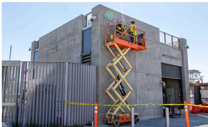
Mariposa Pump Station Improvements Project: Exterior sign installation.
