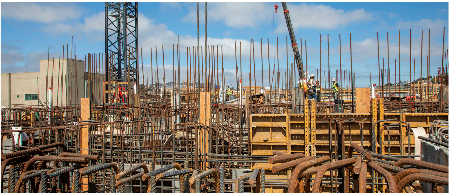
Southeast Treatment Plant, Headworks Facility Project.
