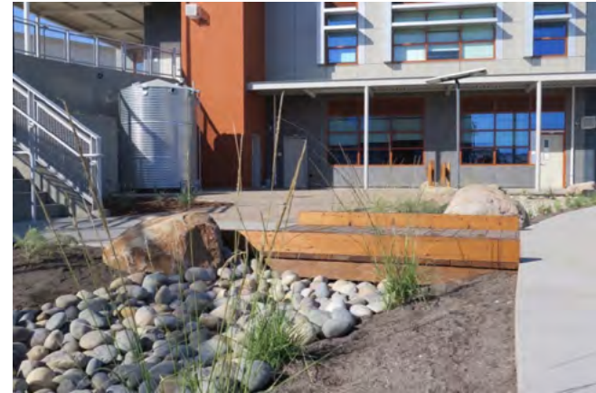
Willie Brown Middle School in San Francisco utilized rainwater harvesting, bioretention, and permeable pavement to comply with the Stormwater Management Ordinance. Photo: Krystal Zamora
