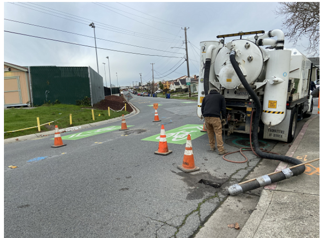
Exploratory Potholing Work
