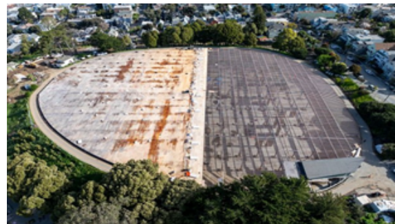
Reservoir Roof Plywood Installation at 50 Percent Completion
