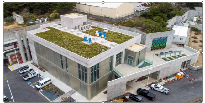
Westside Recycled Water Project - Treatment Facility at Oceanside Plant
