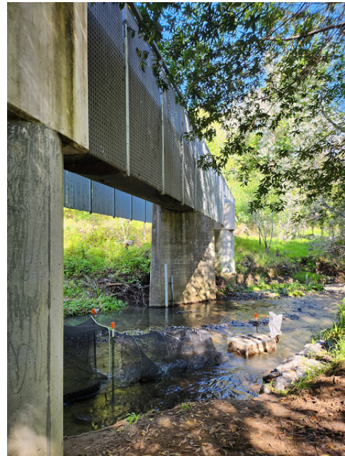
CSPL2 at Creek Crossing
