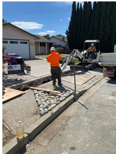
Trenching Sidewalk for Electrical Service Connection to Utility Power at Newark
