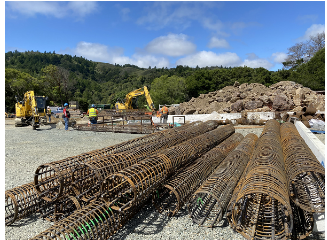
Rebar Cages for Cast in Drilled Hole Piles
