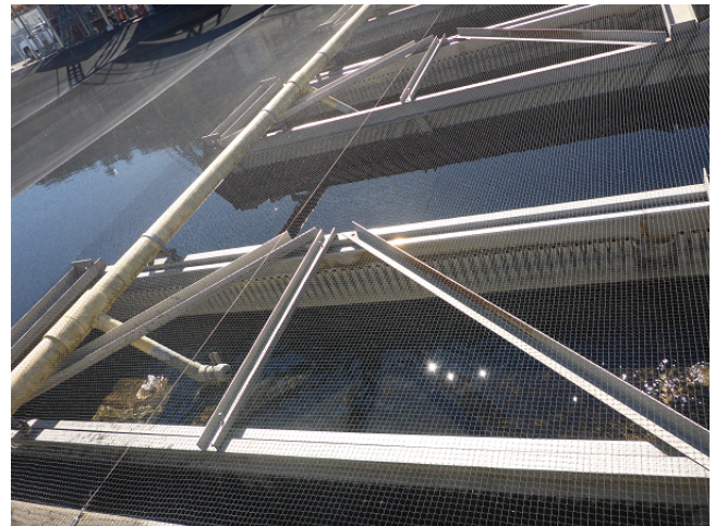
Bird Netting On Sedimentation Basin
