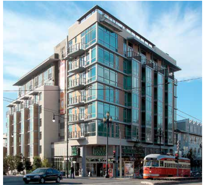
38 Dolores Street (Image courtesy of BAR Architects)
