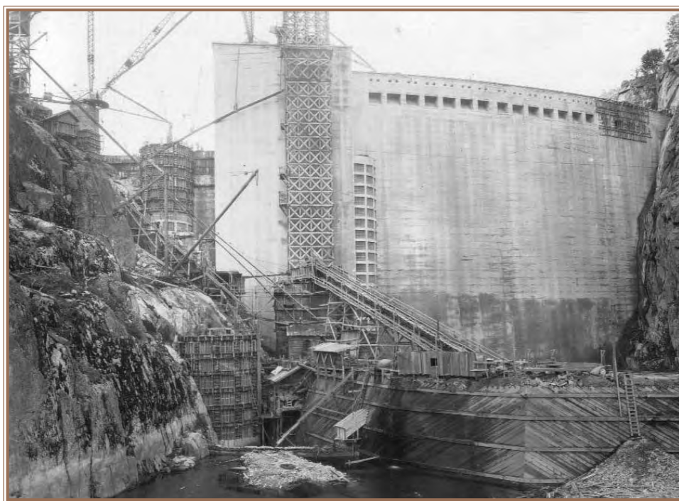
O'Shaughnessy Dam, upstream face 1923
