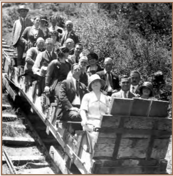
Early Intake Tramway carries visitors to dedicate the dam 1923
