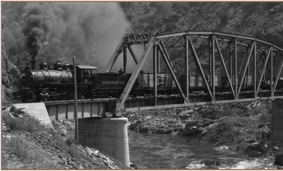
Hetch Hetchy Railroad crossed river gorges to reach the construction site 1919
