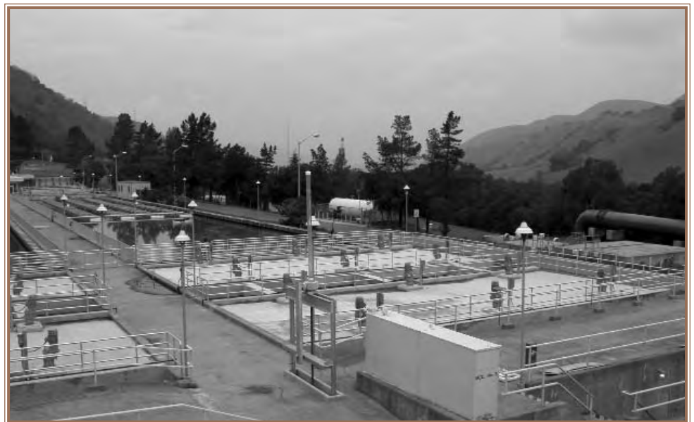
Sunol Valley Water Treatment Plant
