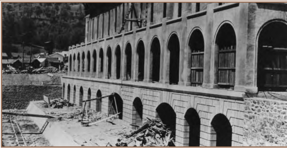
Old Moccasin Powerhouse under construction 1924
