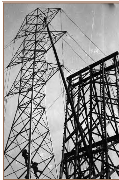
Hetch Hetchy power transmission towers 1924
