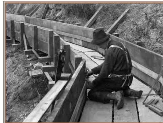
Construction of Stone Dam Flume 1871
