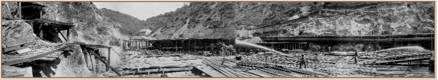
Lower Crystal Springs Dam under construction 1887
