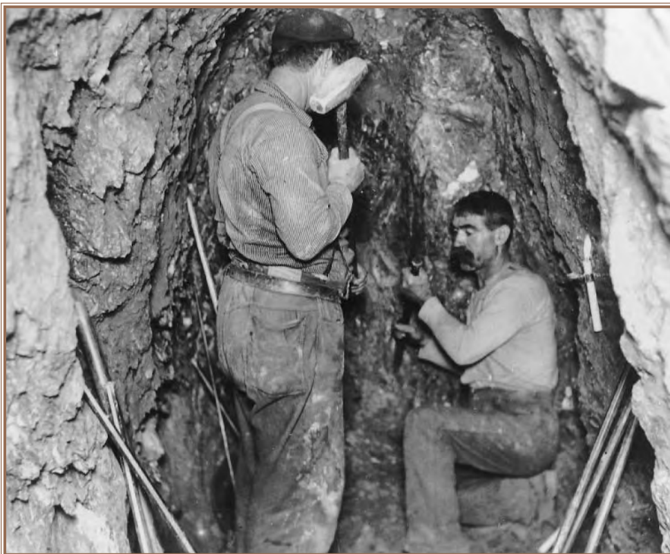
Workers drill Lock's Creek Tunnel 1870
