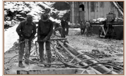
Roughening the crest of O'Shaughnessy Dam 1937
