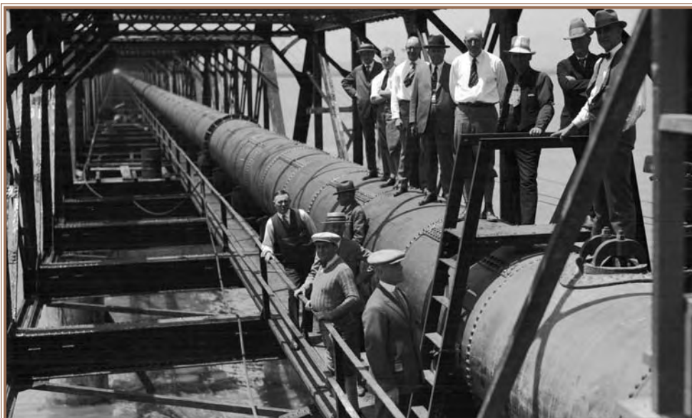
Bay Division Pipeline No. 1 on Trestle Bridge 1925
