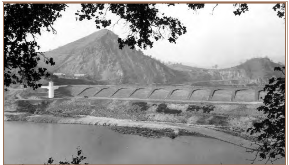
Calaveras Dam and outlet tower 1926
