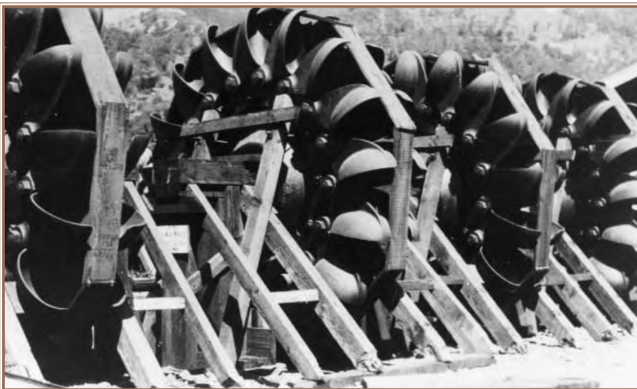
Original Moccasin turbines 1924
