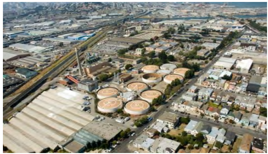
Southeast Treatment Plant
