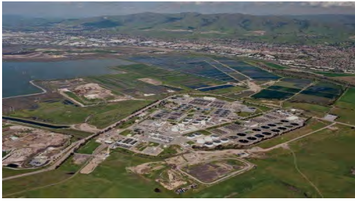
San Jose-Santa Clara Regional Wastewater Facility
