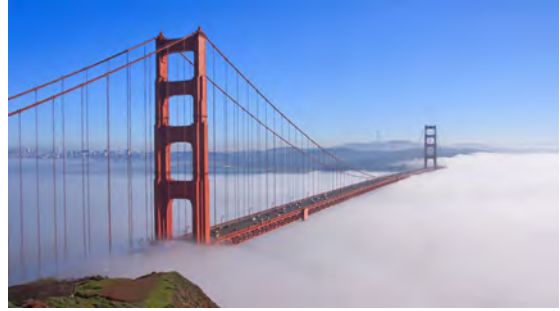
Fog on Golden Gate Bridge
