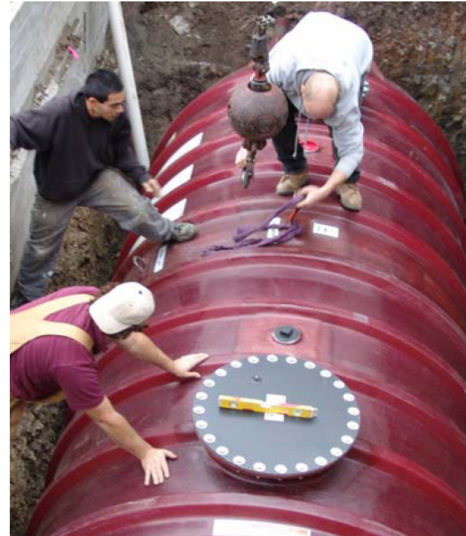
Underground storage tank at a local residence
