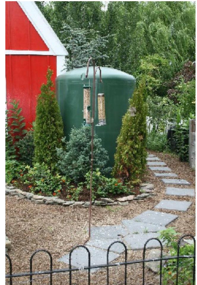
Cistern placement at a residential property
