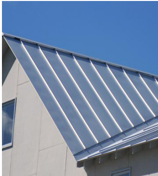
Treated galvanized roof
