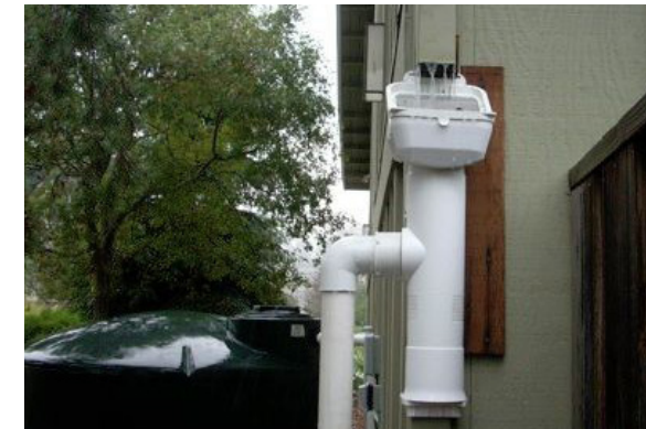
Rain head and First flush diverter www.fubiz.net
