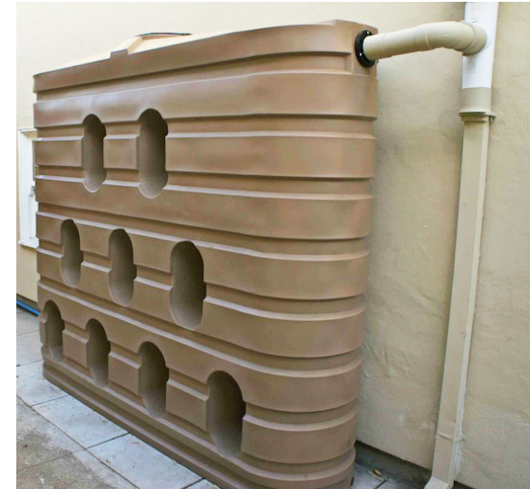
Packaged system with Downspout diverter Photo Courtesy of Oakland Rain Barrel Program
