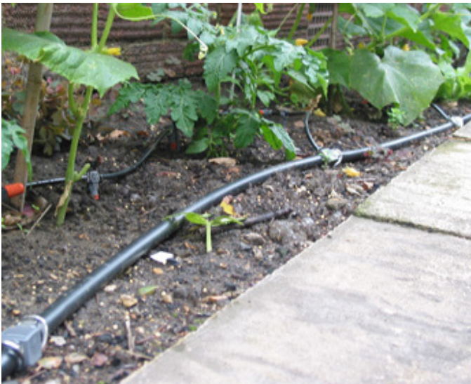
Drip irrigation system in planter
