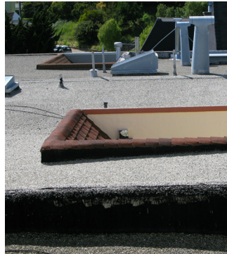
Tar and gravel roof
