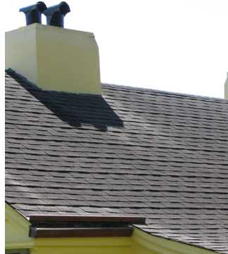
Tile and asphalt shingle roof
