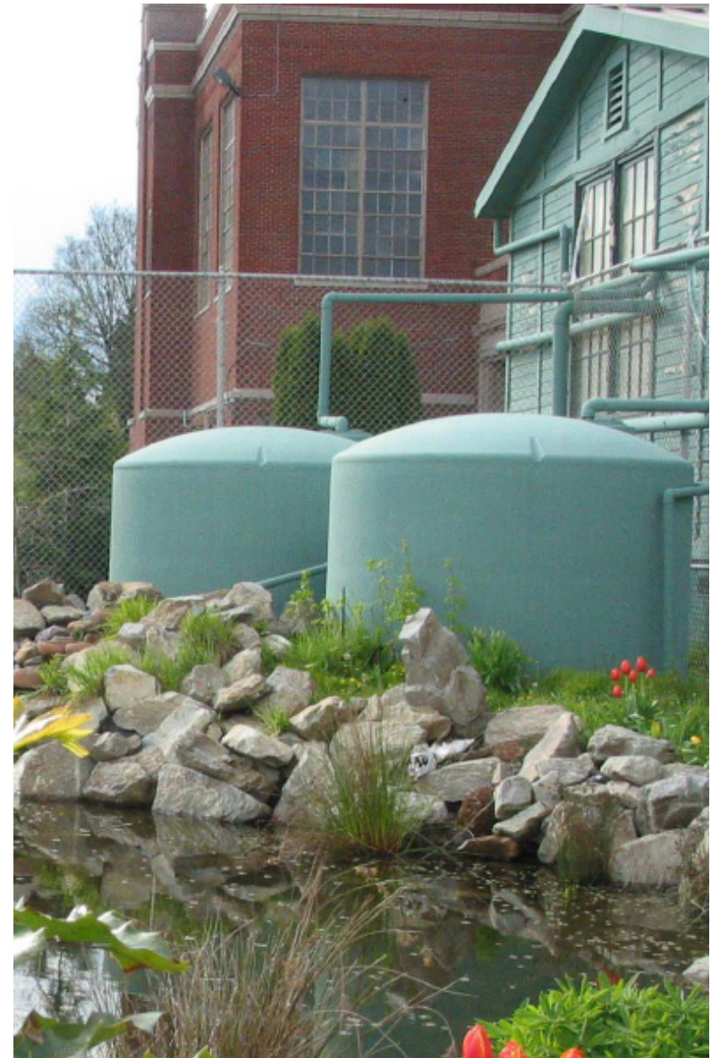
Rainwater harvesting cisterns at a school in Portland, Oregon
