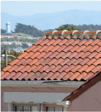
Clay shingle roof
