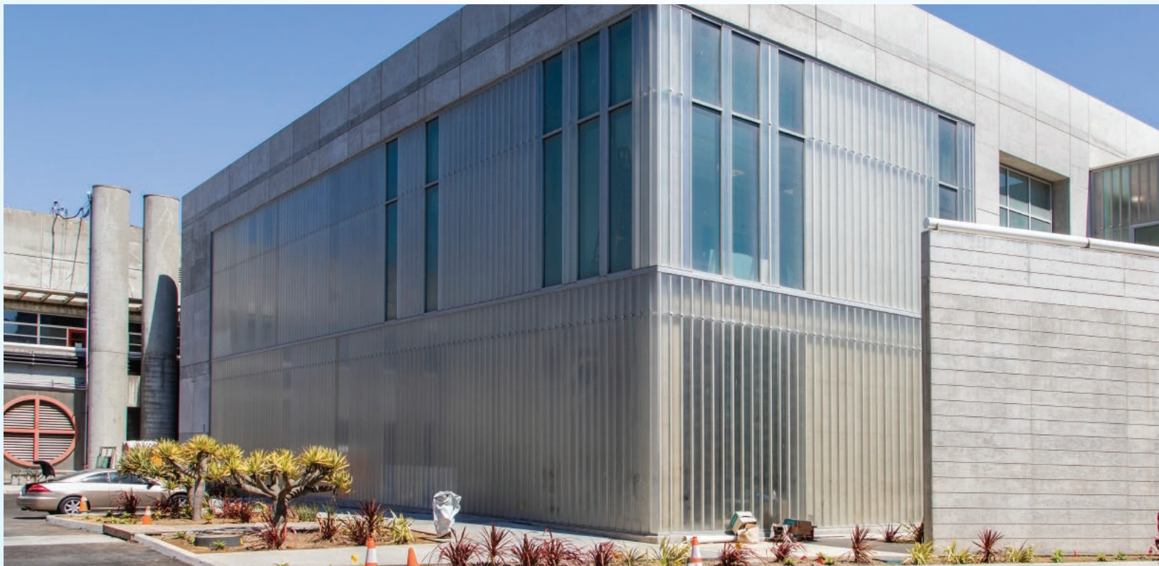
Westside Recycled Water Treatment Facility
