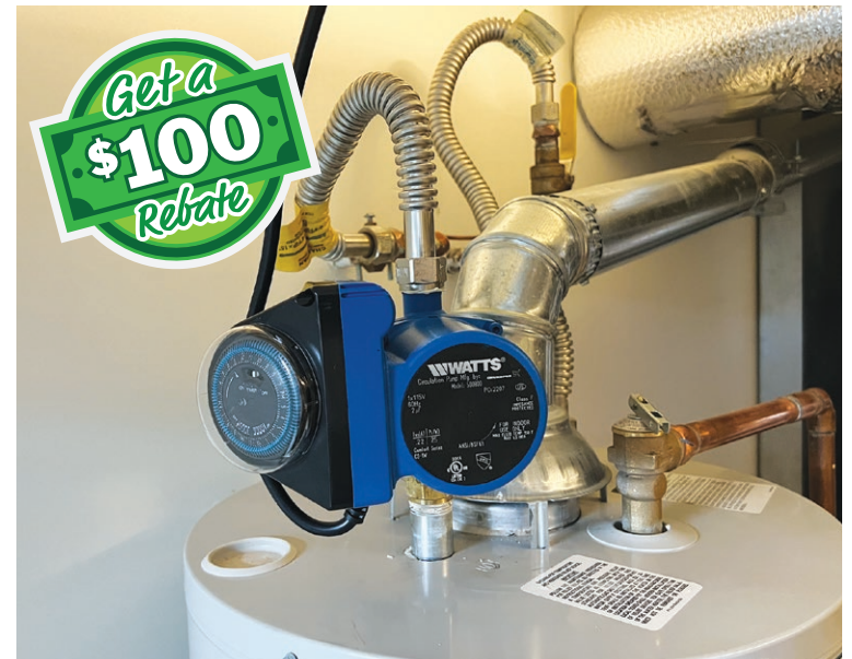
Hot water recirculation pump
