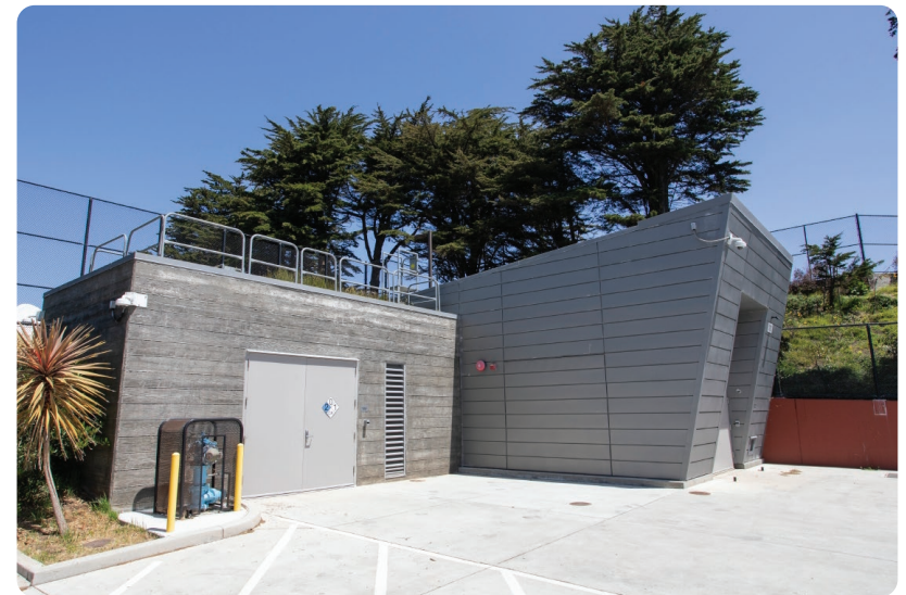
West Sunset Groundwater well station site
