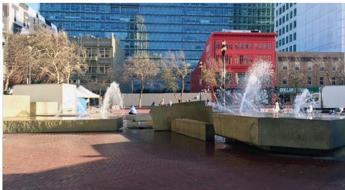
UN Plaza Foundation Drainage Project
