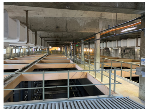
Existing SEP-041 wet-weather primary sedimentation building
