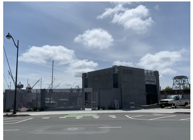
Punchlist items being addressed at Station, including installation of gates and testing of security system
