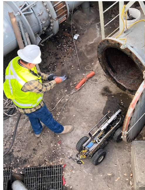
Interior CCTV camera inspection of the discharge manifold
