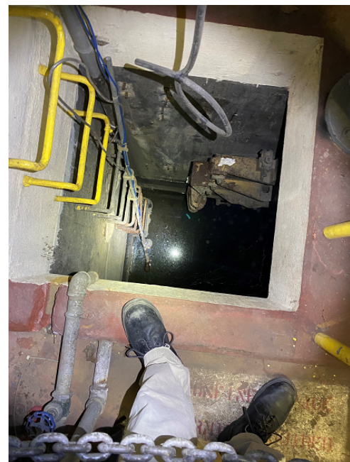
Entrance to Geary Underpass Pump Station
