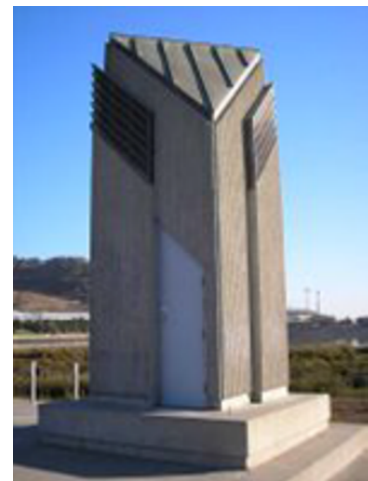
Sunnydale Pump Station
