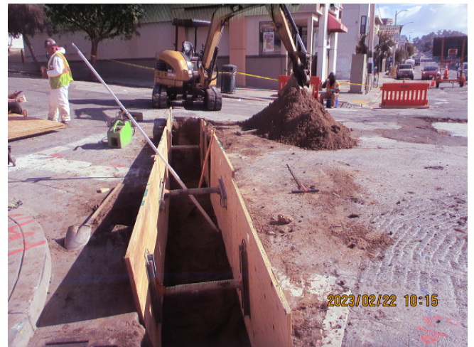
Segment B: 10 inch Culvert Installation NW 22nd Ave
