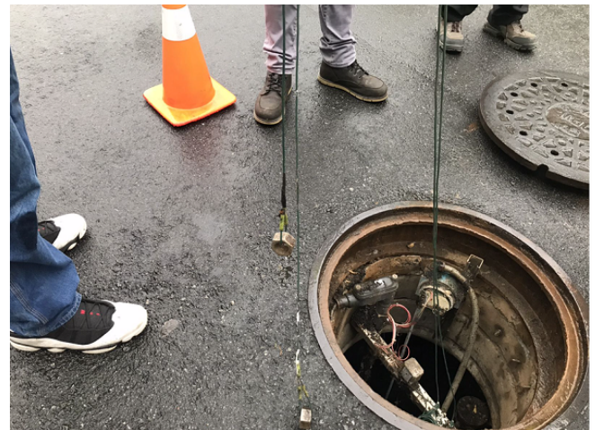
Project team performing field measurements and investigation
