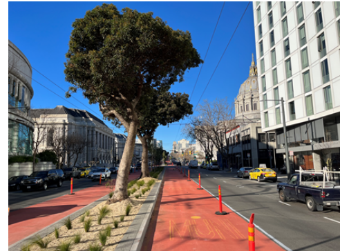
Sewer Completion along Van Ness
