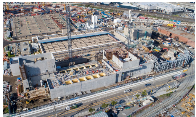
Aerial Drone Photo of the New Headworks Facility
