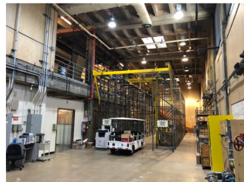
Inside of Bldg SEP 940
