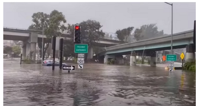
Flooding at the I-280/Hwy 101 interchange at Lower Alemany area, during the rainfall of January 2023
