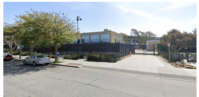
Channel Pump Station
