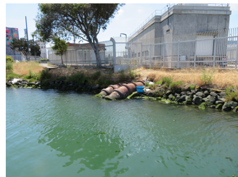
Current pipeline crossing at Islais Creek
