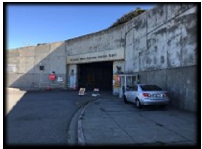
Existing West Vehicle Entrance at Oceanside Water Pollution Control Plant
