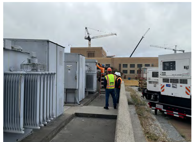
Energization of Substation in Progress
