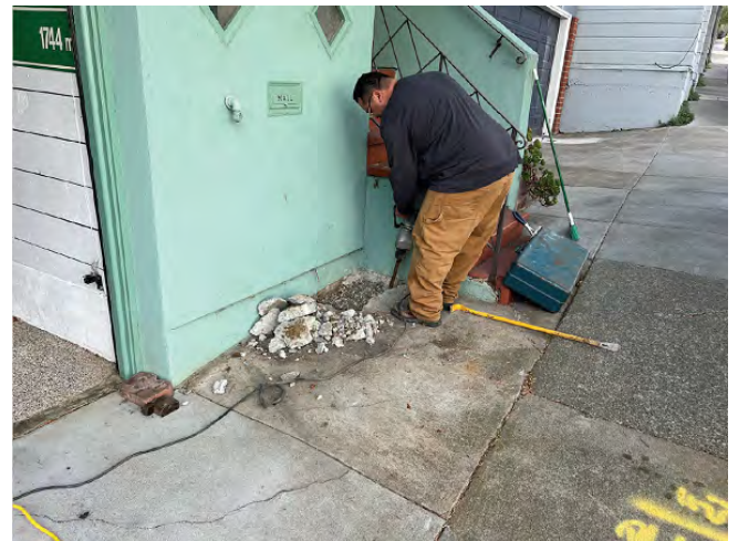
Work in Progress for 37 Chenery Street Floodwater Grant Project.
