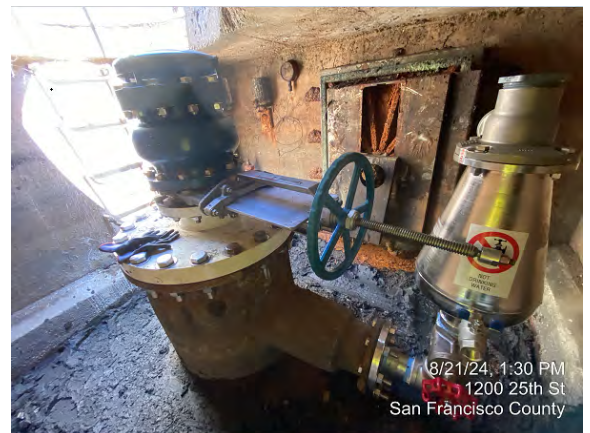
Contract A: Installation of New Air Release Valves
