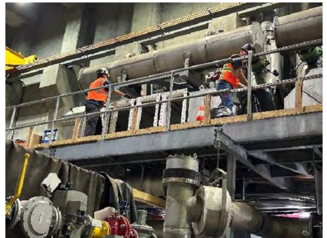
Cogeneration engine exhaust system installation and testing.
