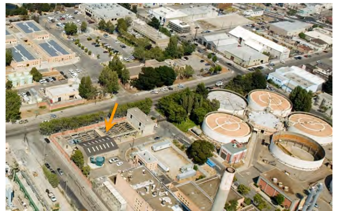
Southeast Plant- Abandoned DAF Units
