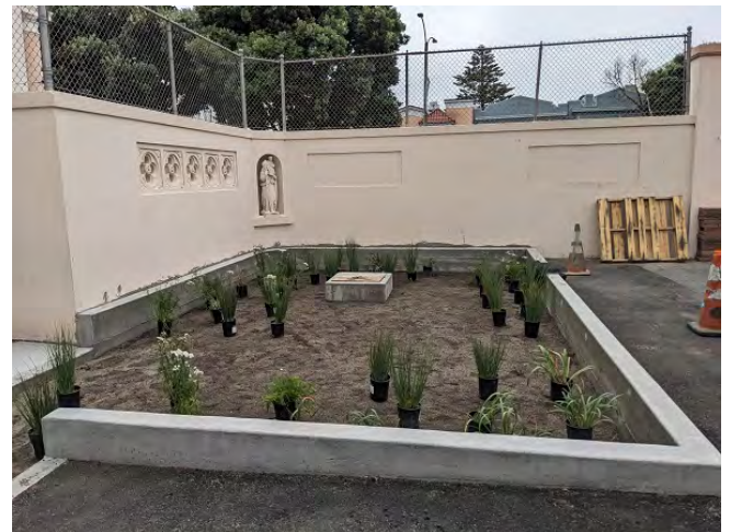
Construction of Rain Garden at St Monica Church and School
