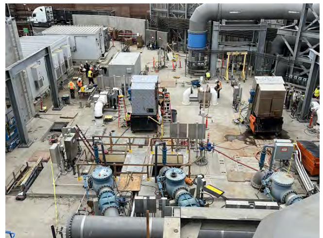
Southeast Pumping Station Construction and Various Forcemains
