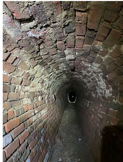
Investigation of 3ft x 5ft Brick Sewer on Folsom Street as Part of Contract WW-719A
