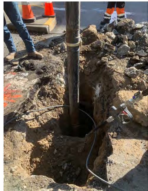
PG&E Pothole Investigation at 6th and Geary
