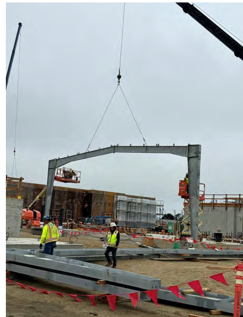
Steel Framework for Biological Nutrient Removal Facility
