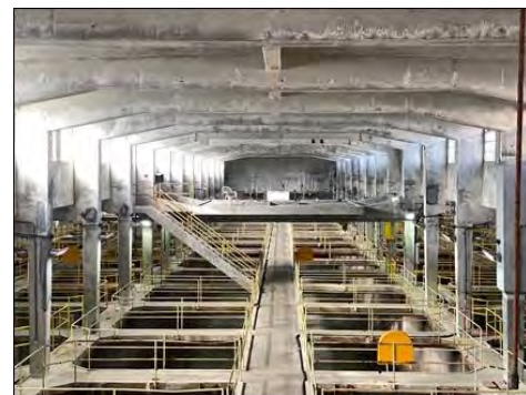
NPF 041 Main Sedimentation Tank Area
