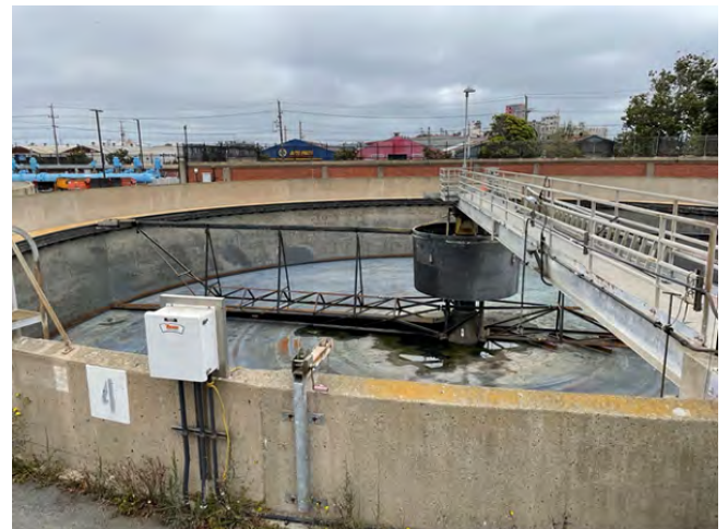
One of the Secondary Clarifiers To be Rehabilitated
