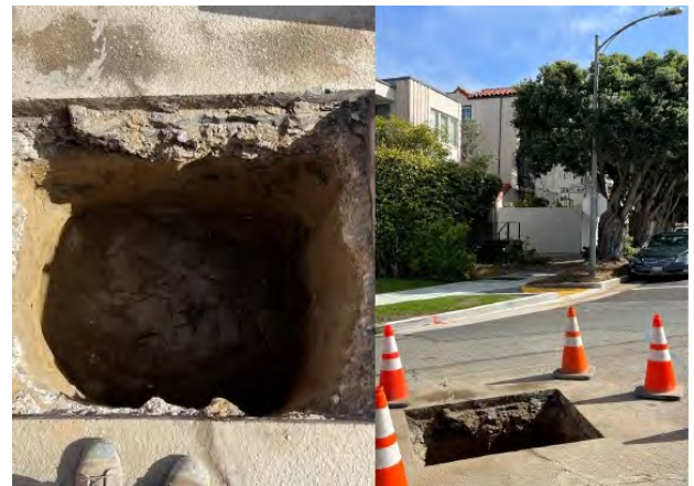
Potholing Investigation for Force Main
