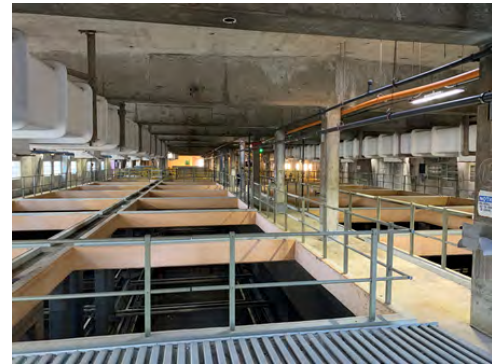
Existing SEP-041 Wet-Weather Primary Sedimentation Building.
