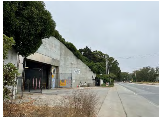
Existing East Vehicle Entrance at OSP
