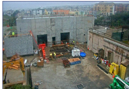
Contractor installing the new cast-in-place concrete Electrical Building as of June 2022.
