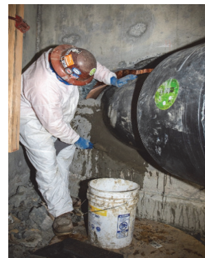
Grouting of new pipe at new underground concrete pipe
