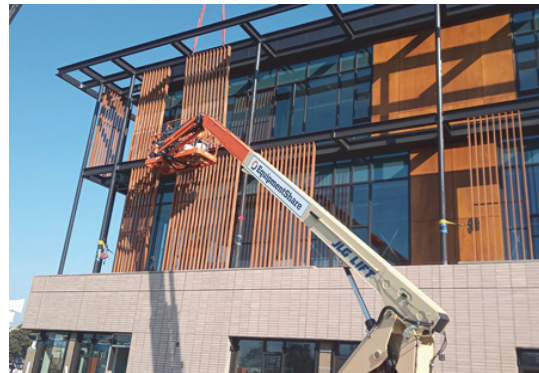
Installation of wood panels and fins on the community center building
