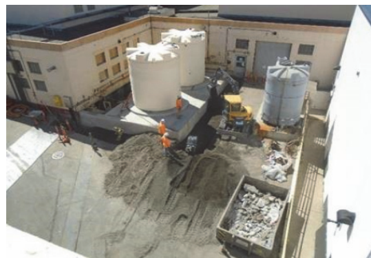
Ferrous Chloride Tanks have being placed on new pads
