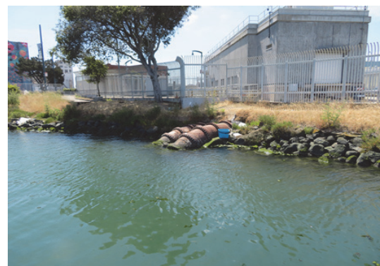
Current pipeline crossing at Islais Creek
