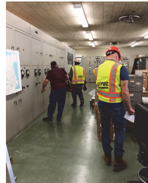
Project team is evaluating removal of existing antiquated electrical equipment.
