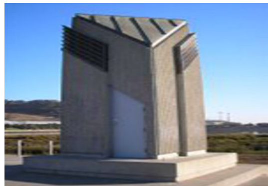
Sunnydale Pump Station
