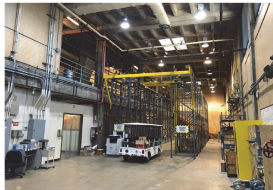
Inside of Bldg SEP 940
