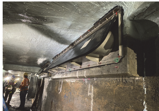
Final walk-through inspection of Sansome St. CSD backflow preventer control valve
