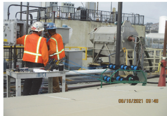
Drum Screen Wire Installation
