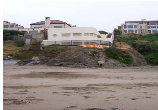
Seacliff No. 2 Pump Station and the CSD 007 discharge location at Baker Beach
