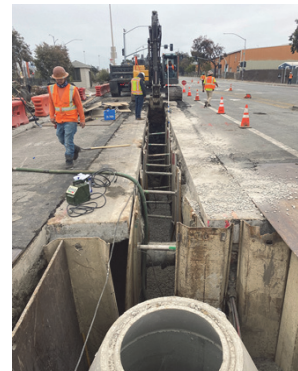
Manhole Installation
