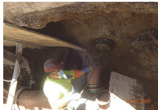
Geary BRT – Sewer Construction
