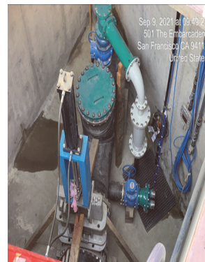
New Finished Vault and Appurtenances
