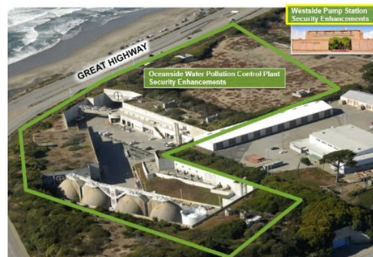
Aerial photo of Oceanside Water Pollution Control Plant and Westside Pump Station Facilities to receive security system enhancements
