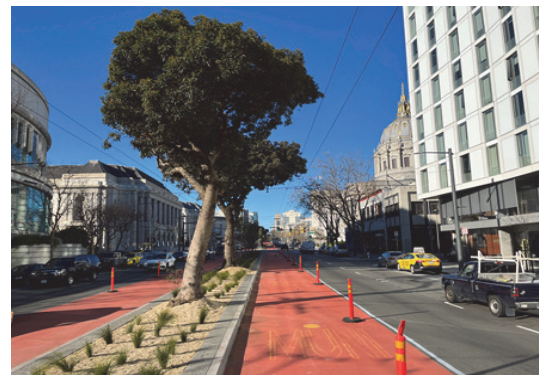
Sewer completion along Van Ness
