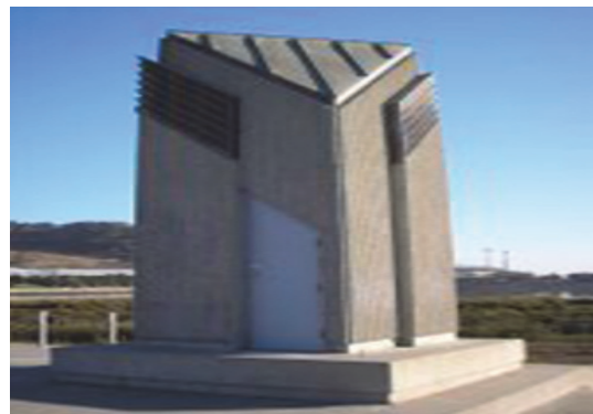
Sunnydale Pump Station
