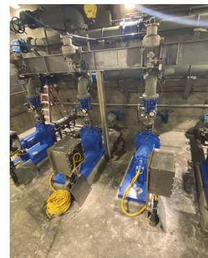
Completed Mechanical Piping
