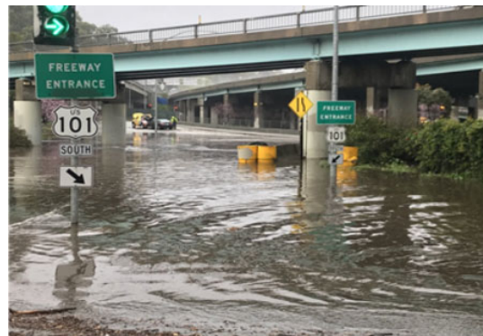
Flooding at the I-280/Hwy 101 interchange at Lower Alemany area, during the rainfall of February 13, 2019
