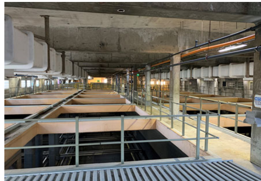
Existing SEP-041 wet-weather primary sedimentation building.
