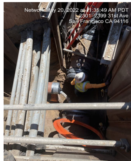
Preparing for manhole construction at 31st and Taraval
