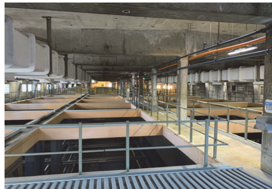
Existing SEP-041 wet-weather primary sedimentation building.
