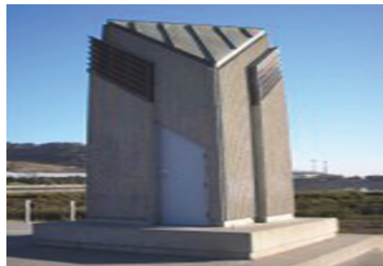
Sunnydale Pump Station
