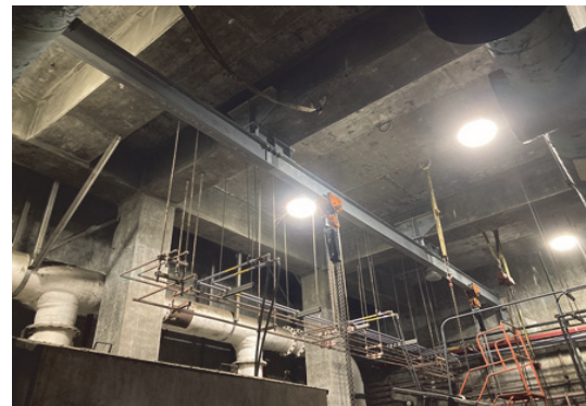
Monorail installation at barscreen room
