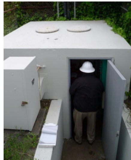
Seacliff Pump Station No.1
