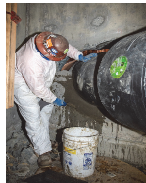
Grouting of new pipe at new underground concrete pipe
