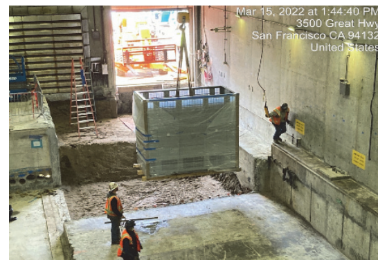
OSP800 Substation 5 medium-voltage electrical transformer delivery (March 2022)
