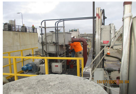
New Rotating Screen Filter / Compactor Installation at SEP 042 Primary Sedimentation Tanks
