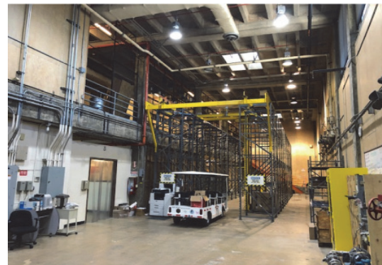
Inside of Bldg SEP 940
