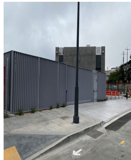
Exterior of the completed Mariposa Pump Station
