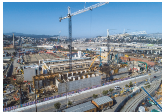
SEP New Headworks Facility – Aerial Drone Footage
