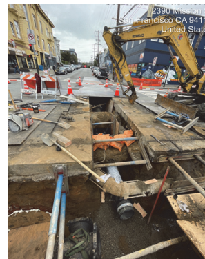
AWSS Construction at the intersection of 20th and Mission Streets
