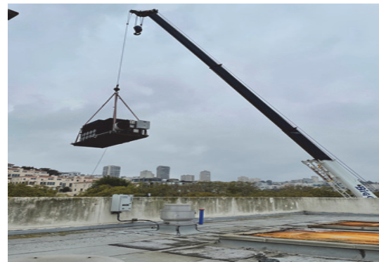
Removal of existing Odor Control Unit (OCU)
