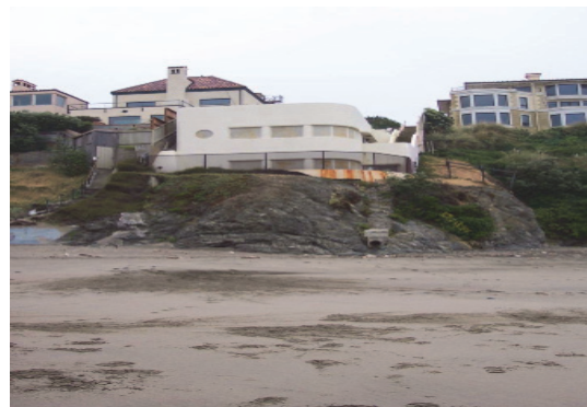
Seacliff No. 2 Pump Station and the CSD 007 discharge location at Baker Beach
