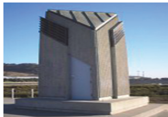
Sunnydale Pump Station
