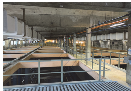
Existing SEP-041 wet-weather primary sedimentation building.
