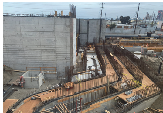
Hydraulic Channels and portion of Grit Tank Area Structure
