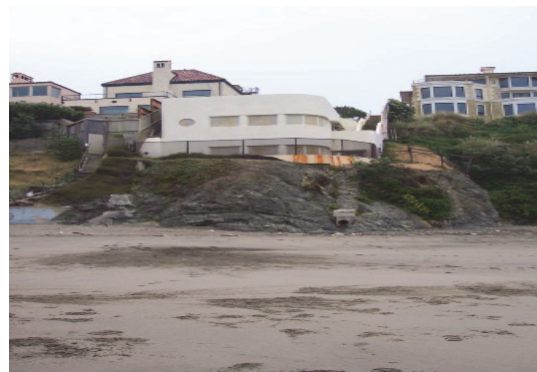
Seacliff No. 2 Pump Station and the CSD 007 discharge location at Baker Beach
