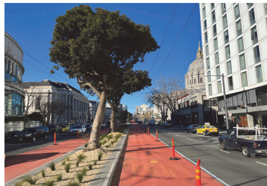
Sewer completion along Van Ness
