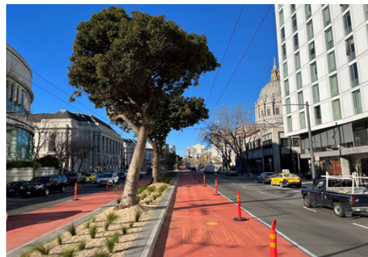
Sewer Completion along Van Ness
