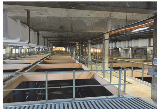
Existing SEP-041 wet-weather primary sedimentation building.
