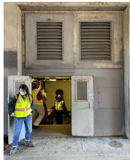
Entrance to Geary Underpass Pump Station
