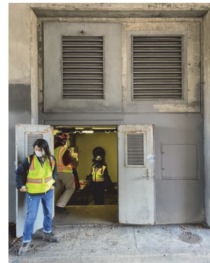
Entrance to Geary Underpass Pump Station
