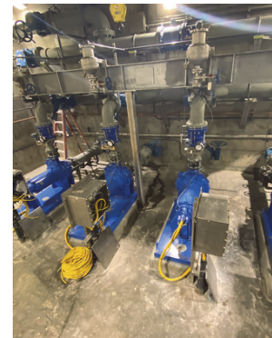
Completed Mechanical Piping
