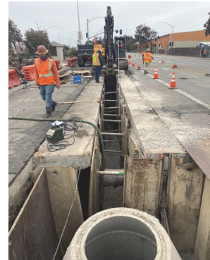
Manhole Installation
