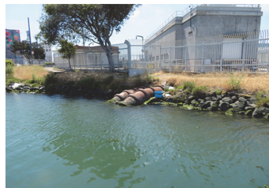
Current pipeline crossing at Islais Creek
