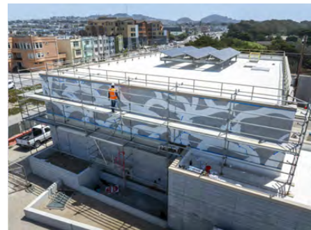
Public Art Mural Installation on New Electrical Building
