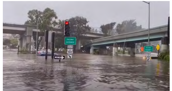
Flooding at the I-280/Hwy 101 Interchange at Lower Alemany Area, During the Rainfall of January 2023
