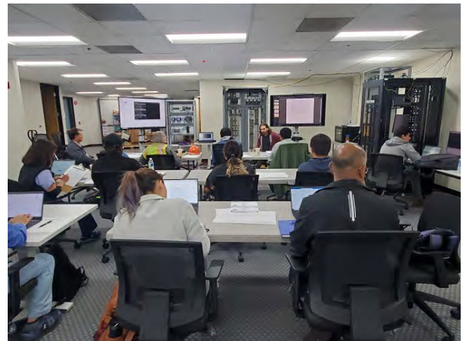
Northshore Pump Station DCS Hardware Operational Readiness Test
