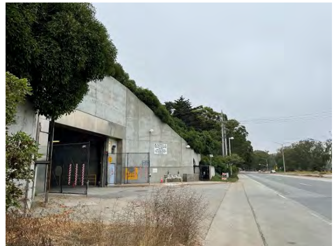
Existing East Vehicle Entrance at OSP
