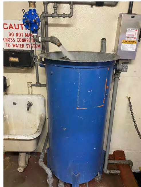
Water Connection Field Testing
