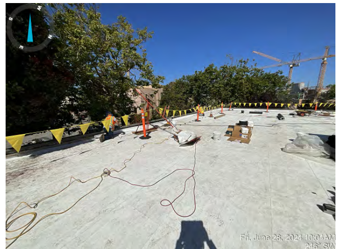
SEP HVAC Work at SEP 260 and Door Replacement Work at SEP 040/041
