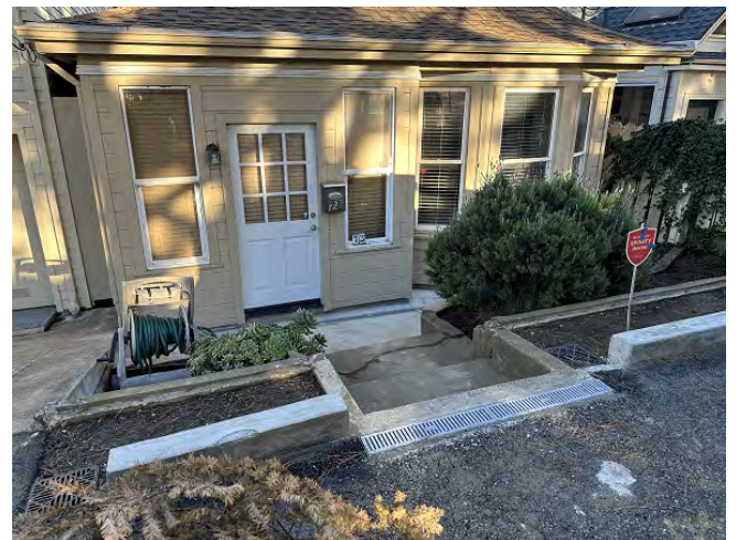
Completed Floodwater Grant project at 73 Mansfield St.
