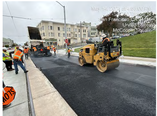
Segment B Paving Taraval Street
