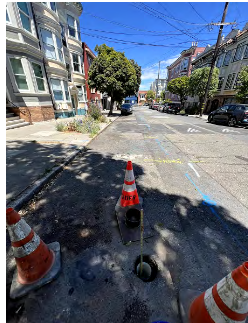
Soil infiltration testing on Cumberland Street.
