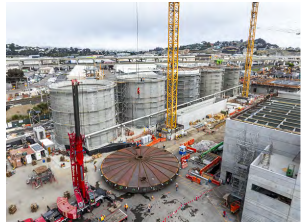
Preparation for Installing Digester Cover
