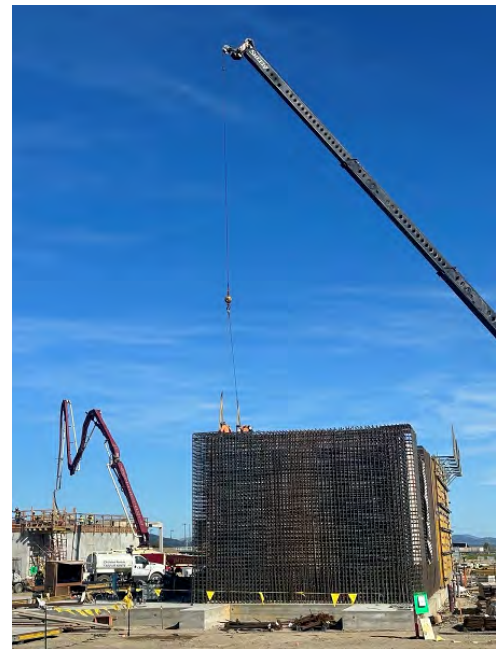
Construction of Solids Handling Building
