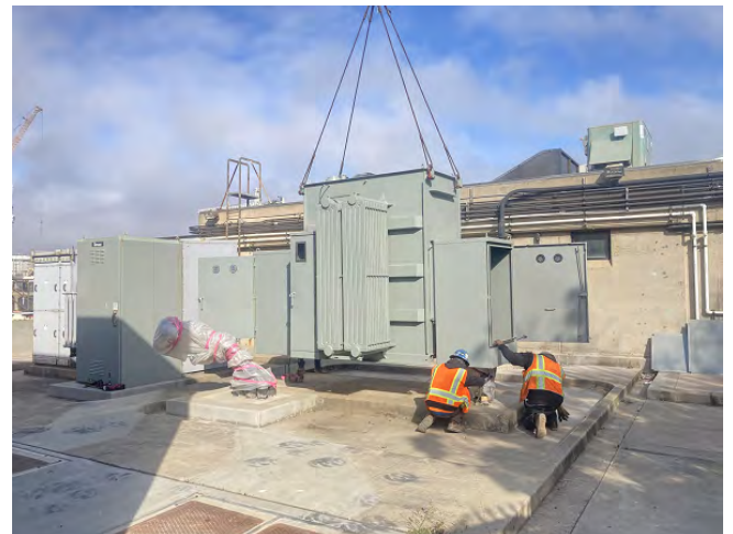
Installation of New Substation 3A
