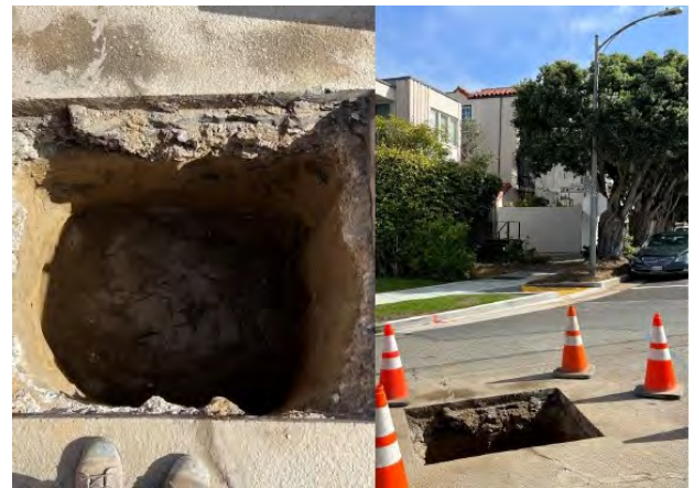
Potholing Investigation for Force Main
