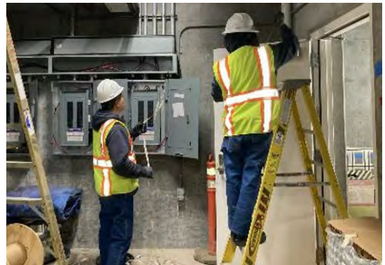
Contractor Installing New Wiring in Building 800
