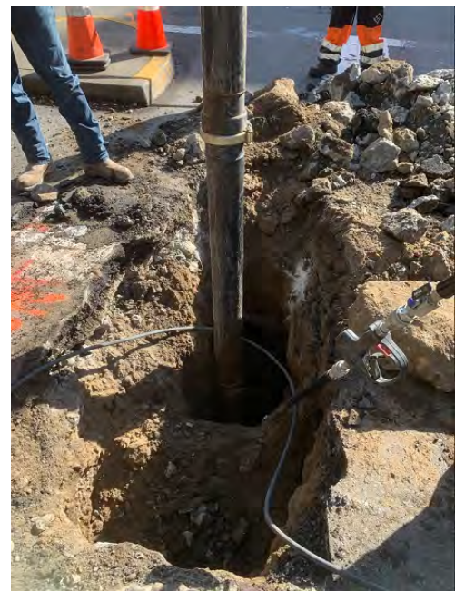
PG&E Pothole Investigation at 6th and Geary
