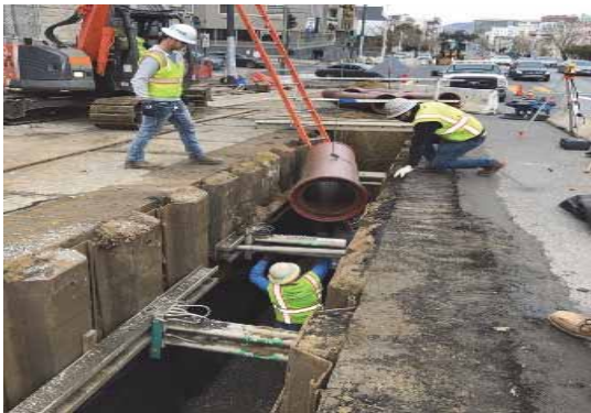
Sewer construction along Van Ness
