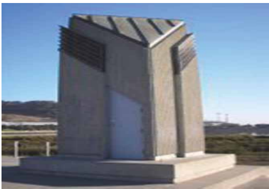
Sunnydale Pump Station
