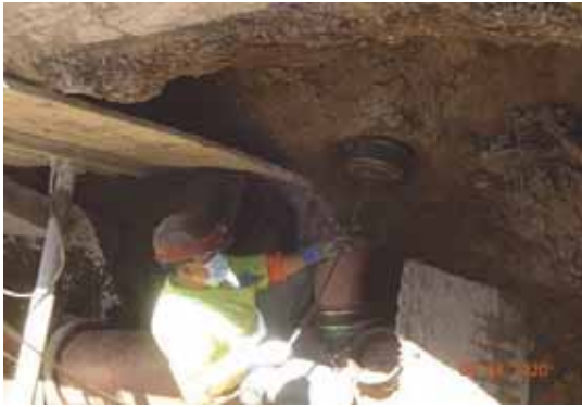
Geary BRT – Sewer Construction
