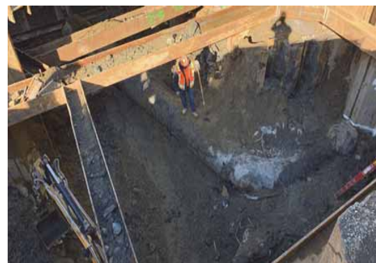
Excavated Existing Force Main
