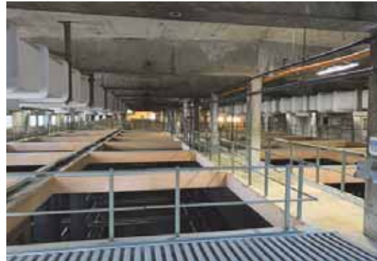
Existing SEP-041 wet-weather primary sedimentation building.
