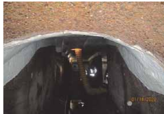
Looking into repaired 5th St. CSD discharge pipe
