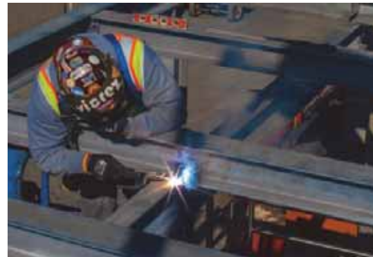
Canopy Installation at South of SEP 042
