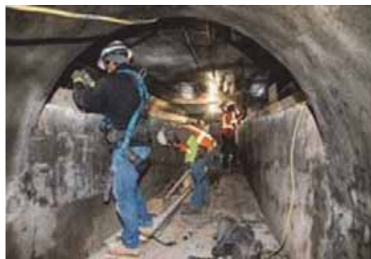
Rehabilitation work at Griffith Combined Sewer Discharge structure
