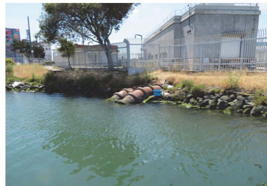
Current pipeline crossing at Islais Creek
