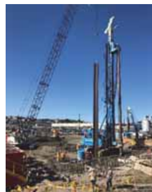
Installation of Foundation Wall for Solids Pretreatment Facility
