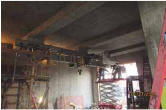
Bridge Crane Installation
