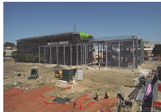
Construction proceeding with building envelope.
