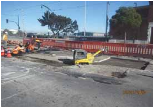
WW-696 Backfill After 12-inch Water Line Relocation on 3rd St.
