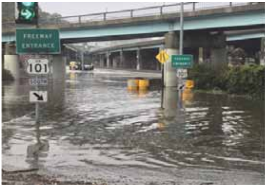
Flooding at the I-280/Hwy 101 interchange at Lower Alemany area, during the rainfall of February 13, 2019
