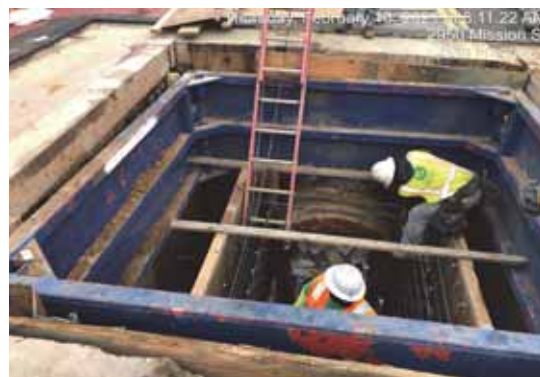
Manhole reconstruction work in progress
