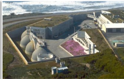
Oceanside Treatment Plant
