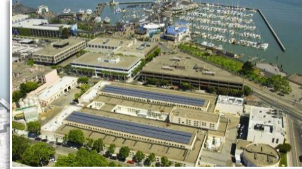
North Point Wet Weather Facility
