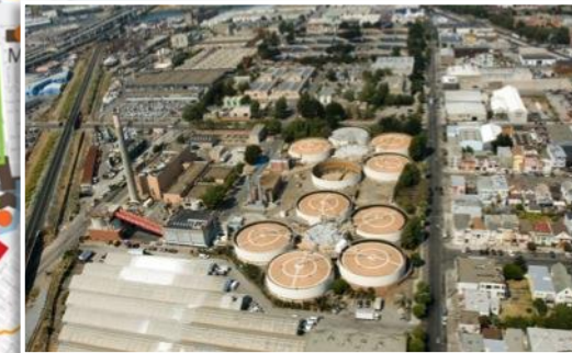
Southeast Treatment Plant
