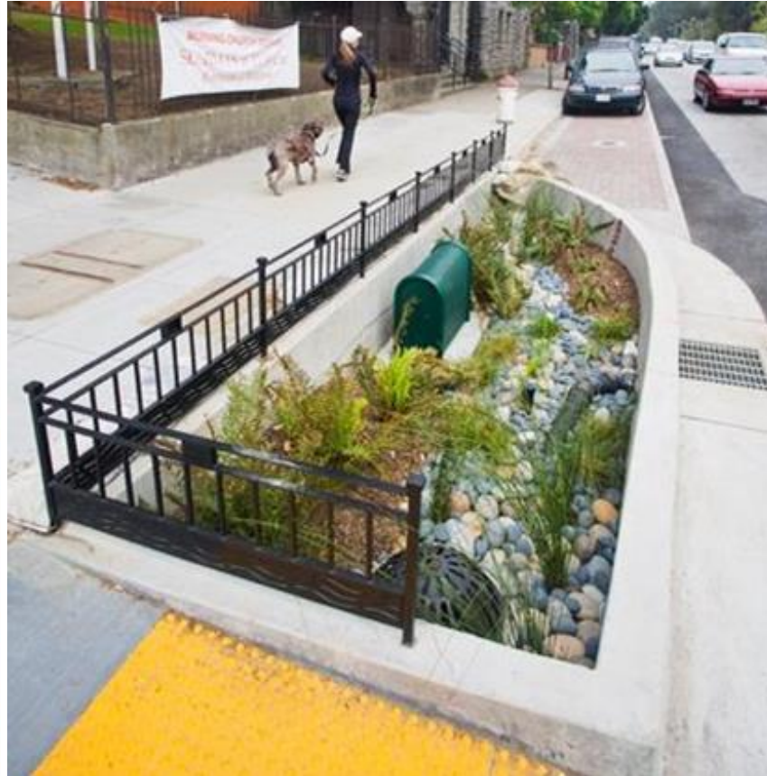
Innovative Stormwater Management Solutions
