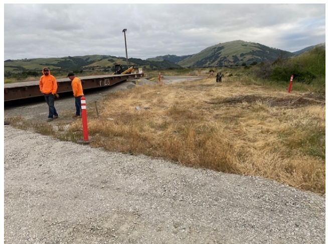
Demobilization of railcar bridge over DWR pipeline
