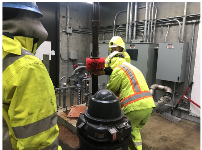
Well brushing at Colma BART Well Facility as part of Phase 2A (Contract C) WD-2878A
