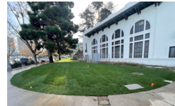
AWSS Pump Station No. 2 Improvements
