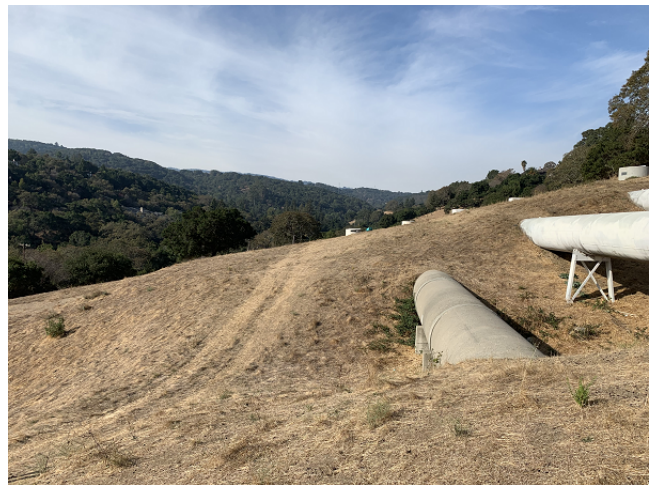
Alignment of BDPL1-5 through Rolling Terrain
