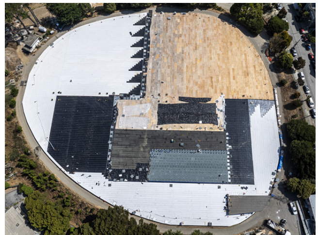
Reservoir Roof Membrane Installation approaching 50% Completion
