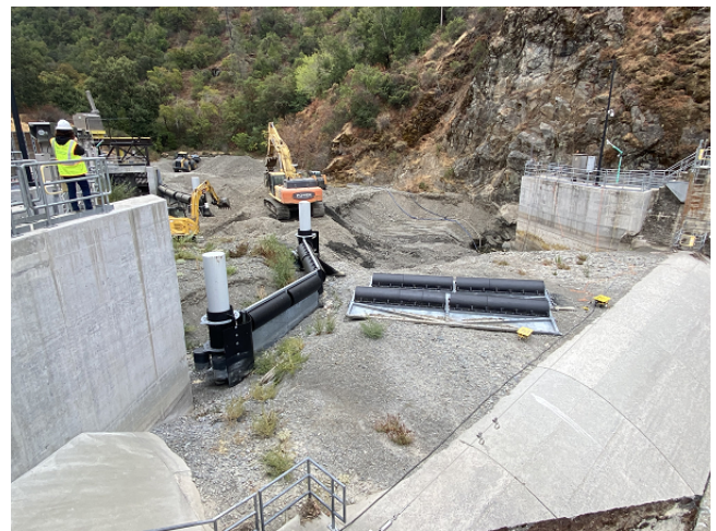
Forebay Sediment Excavation
