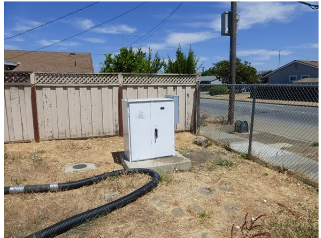
Corrosion on Existing Air Scour Pipeline at the Sunol Valley Water Treatment Plant
