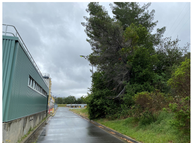
Access Road at Chemical Tanks and Building at the Sunol Valley Water Treatment Plant
