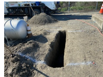
Utility Potholing Work
