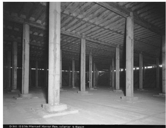
Interior of Merced Manor Reservoir During Construction in 1936
