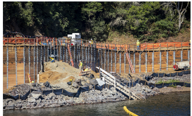
Excavation and Lagging
