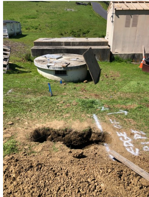
Utility Potholing Work
