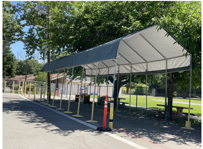
Sunol Glen School Shade Structure to be Removed for Construction
