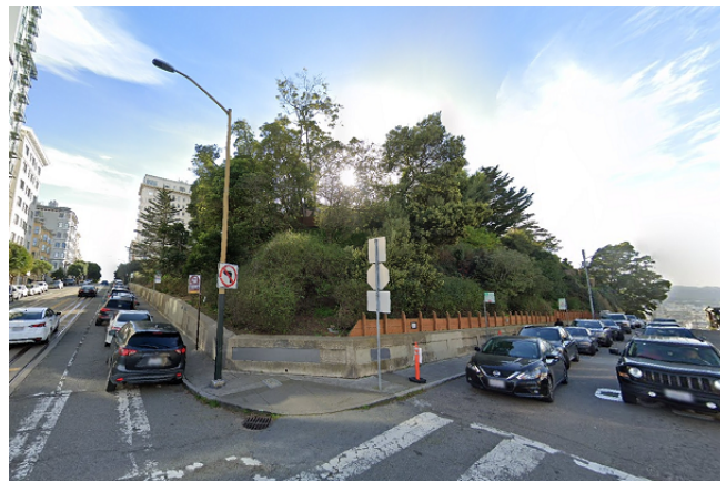
Wooden Retaining Wall (2016) at Lombard Reservoir North Slope
