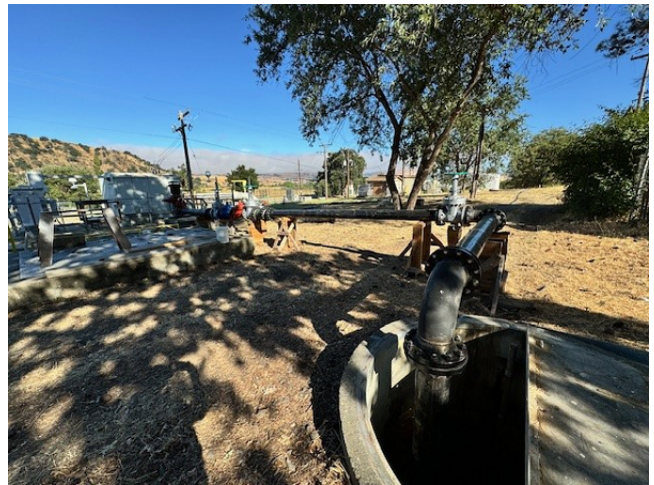
Turner Dam Bypass Pipeline Installation
