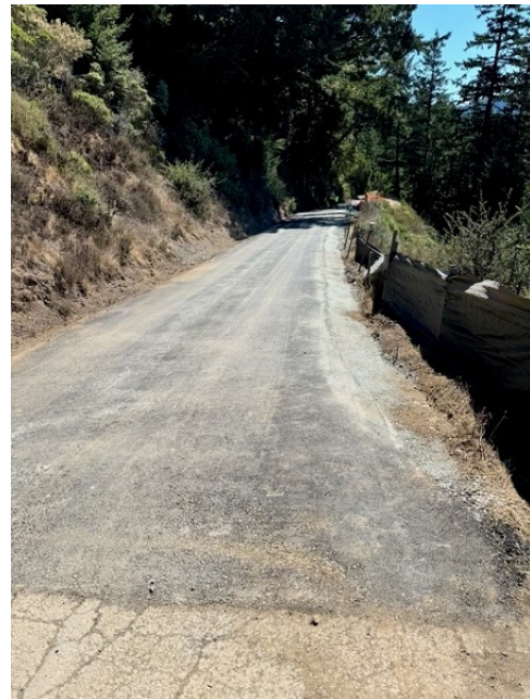
Pilarcitos Dam Access Road
