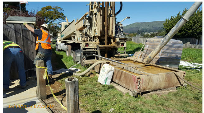
Drill Rig Photo
