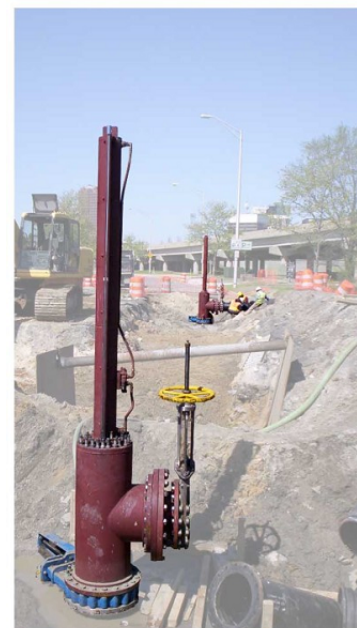
Typical Hot Tap for Line Stop Insertion
