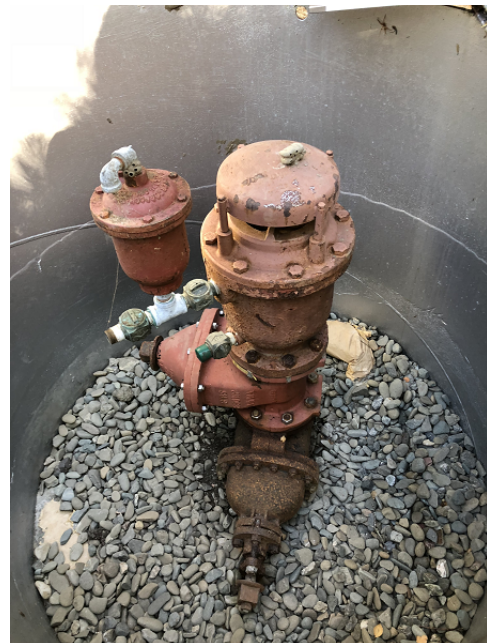
Typical Appurtenance to be Upgraded
