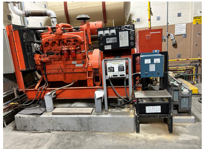
Existing Diesel Emergency Generator being Replaced with New Propane Generator to Backup SAPS Facility
