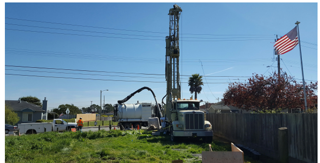
Typical Anode Well Drilling
