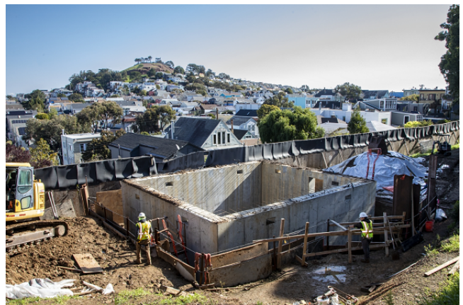
The valve control vault construction
