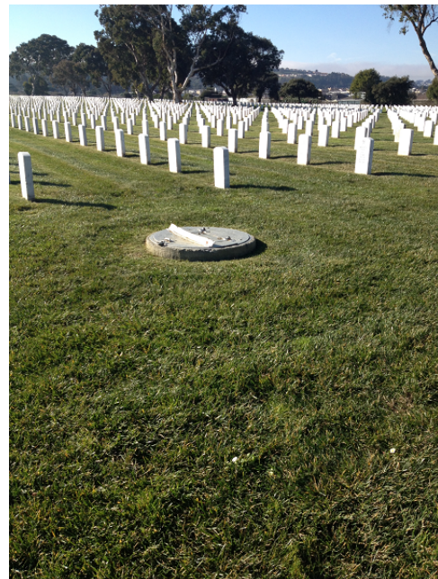
Typical Appurtenance to be Upgraded
