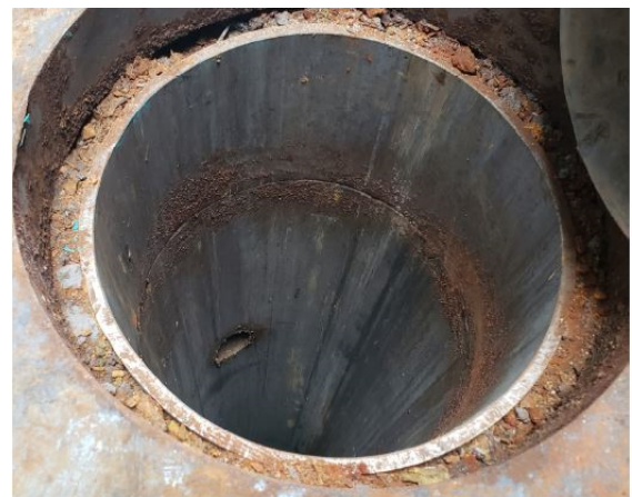
Typical Well Casing
