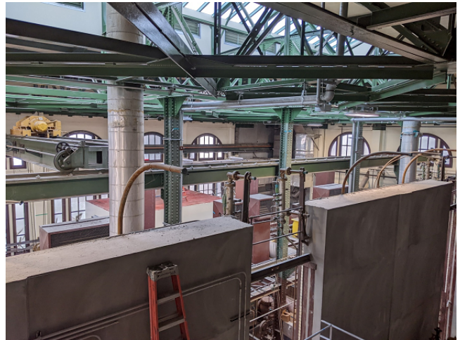
Roof installation of Pump Station No. 2
