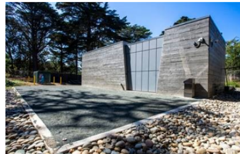
North Lake Well Station
