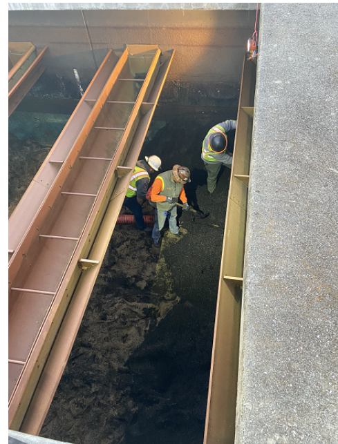
Removal of Filter Media
