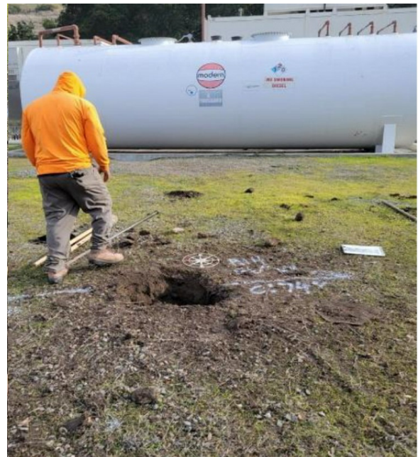
Utility Exploration at San Antonio Pump Station
