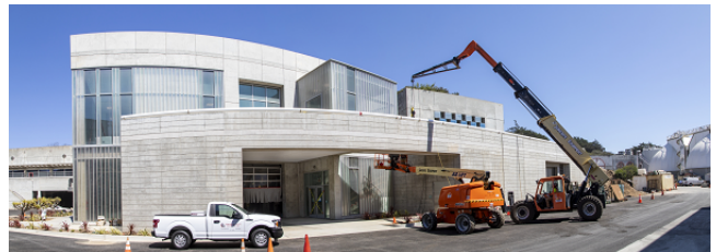
Exterior of Buildings 580 and 581
