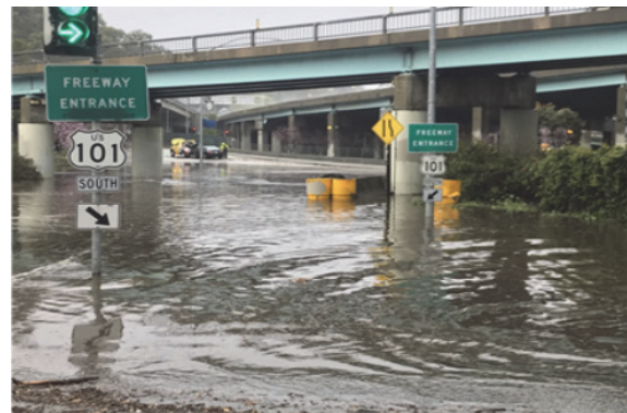
Flooding at the I-280/Hwy 101 interchange at Lower Alemany area, during the rainfall of February 13, 2019
