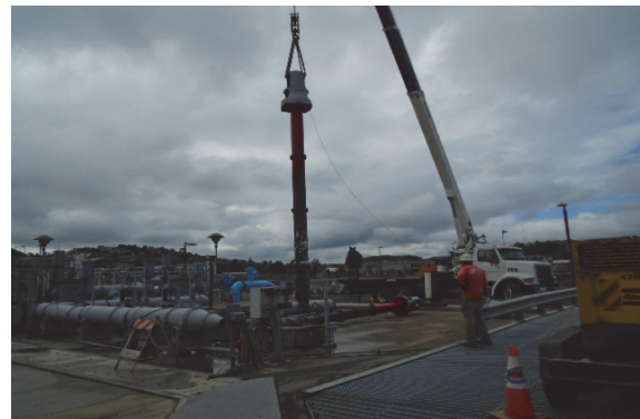
Demo Abandoned Sump Pump System
