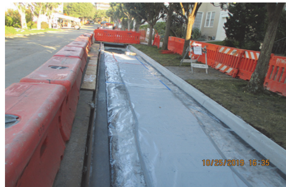
Pervious concrete installation on the south side of Sea Cliff Ave.
