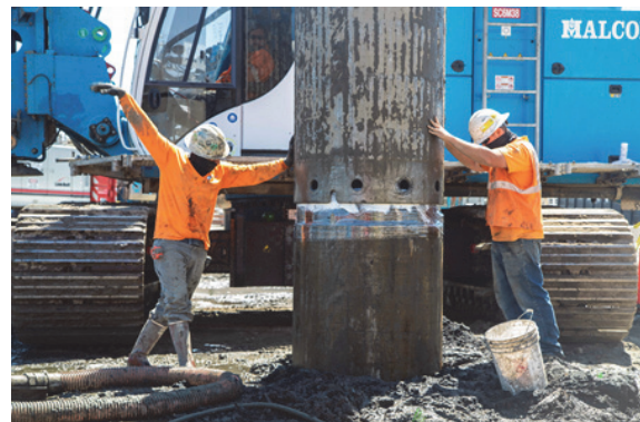
Drilled Piers/ Aligning and installing 20' long casing sections
