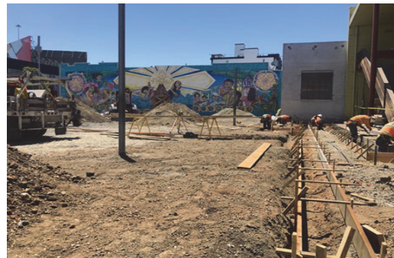
View of Bessie Carmichael Middle School during construction
