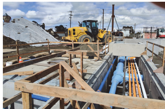
No. 3 Water Line in Trench C to Headworks/BDFP/SEP-042/BFS
