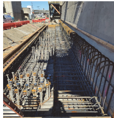
Seismic Piles on Southside
