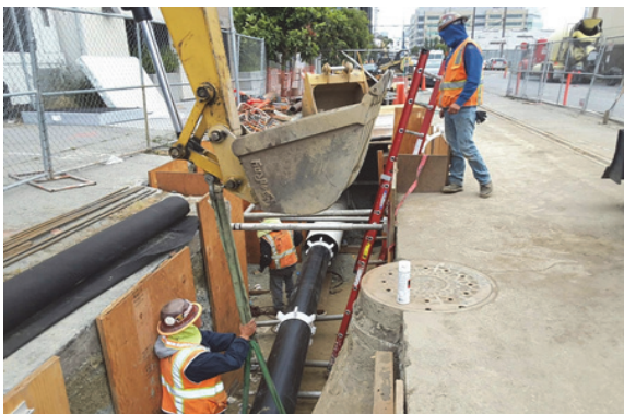
Insertion of the HDPE Force Main
