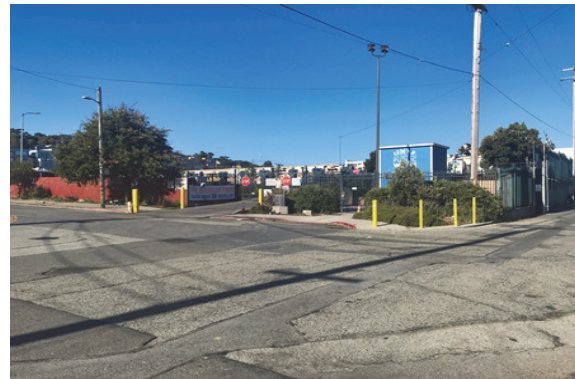
KM MTBM Receiving Area
