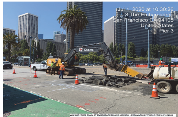
WW-687: Excavating Pit Hole for Slip-Lining
