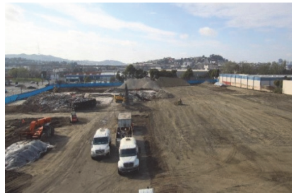
1550 Evans Demolition completion
