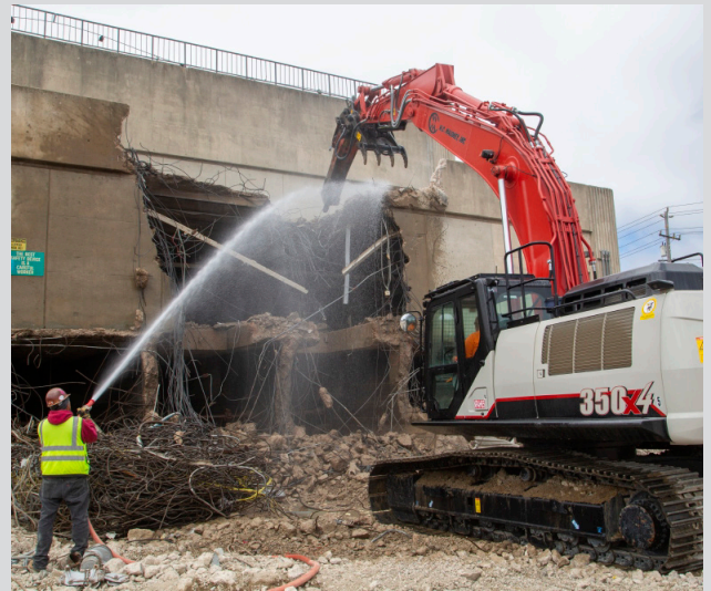
Demolition of existing Headworks Building at Southeast Treatment Plant
