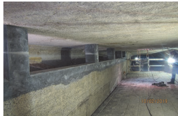
Concrete weir repair at 6th St. CSD
