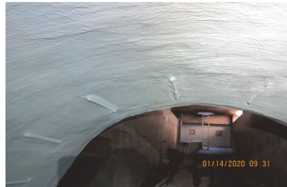
Concrete rehabilitation and protective coating at 5th St CSD
