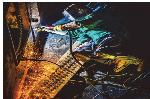
Scope II.A (Bruce Flynn Station Improvements)
