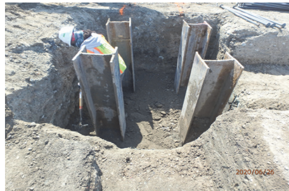
Pile driving completed
