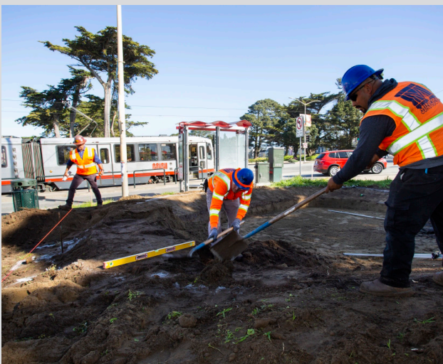
Sunset Boulevard Greenway: Excavation for rain gardens, Sunset Boulevard & Judah Street.
