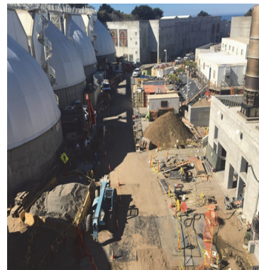
WW-639 Contractor activities including installing site underground utilities on-going
