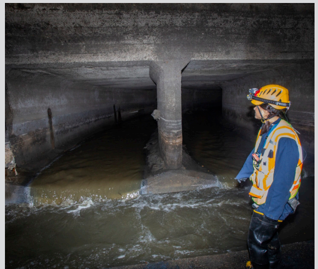
Survey, Scan and Inspection of a Combined Sewer Overflow Structure
