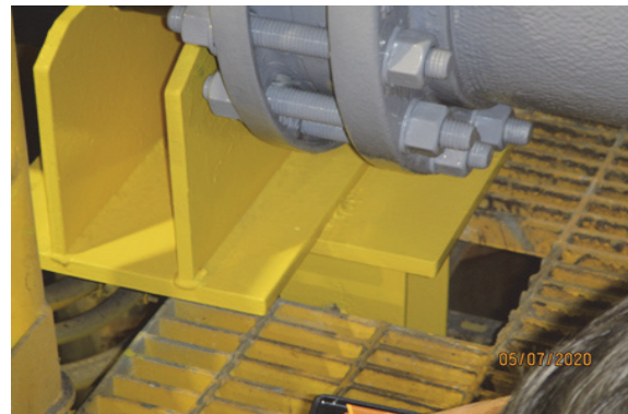
WW-651: Address Vibration in Manifold Room
