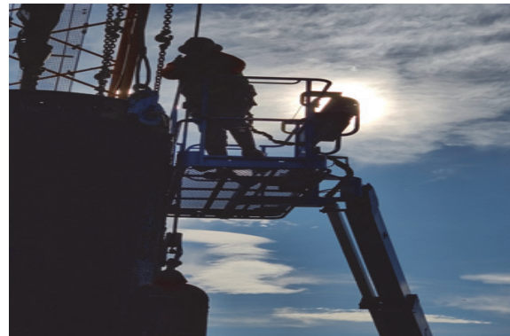
5' Diameter Drill Pier Installation
