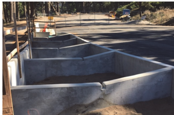
Bioretention planter at north side of El Camino del Mar
