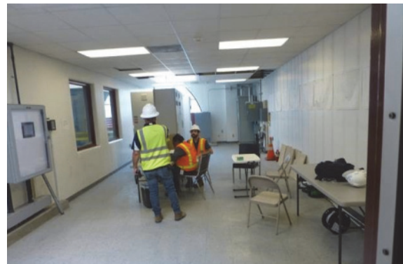
DCS Contractor Testing Control Loops at Bruce Flynn Pump Station
