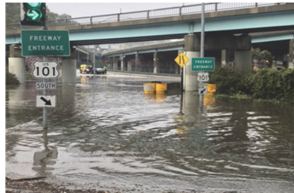
Flooding at the I-280/Hwy 101 interchange at Lower Alemany area, during the rainfall of February 13, 2019
