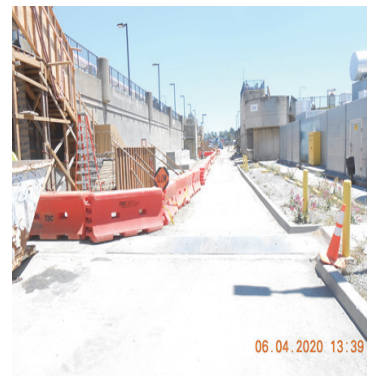
SEP 042 Seismic Support Construction
