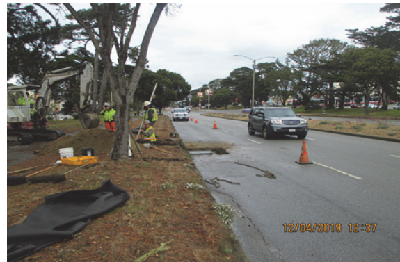
Drain inlet installation on Sunset Blvd. between Judah and Kirkham St.
