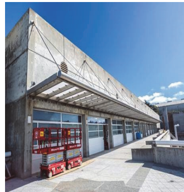
WW-606R2 Building 930 Upper Awning substantially complete in August 2019.
