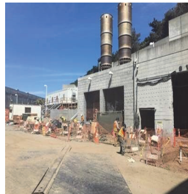
WW-639 Contractor installing yard underground utilities and infilling openings at Building 820
