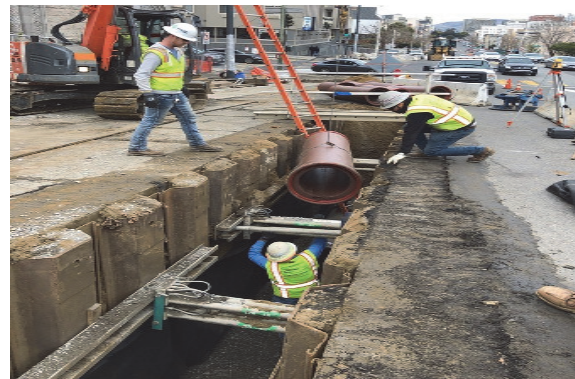
Sewer construction along Van Ness
