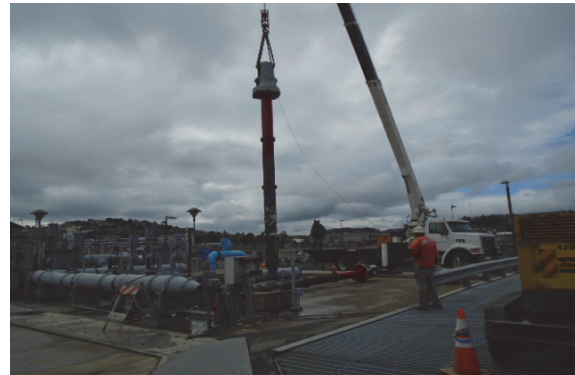
Demo Abandoned Sump Pump System
