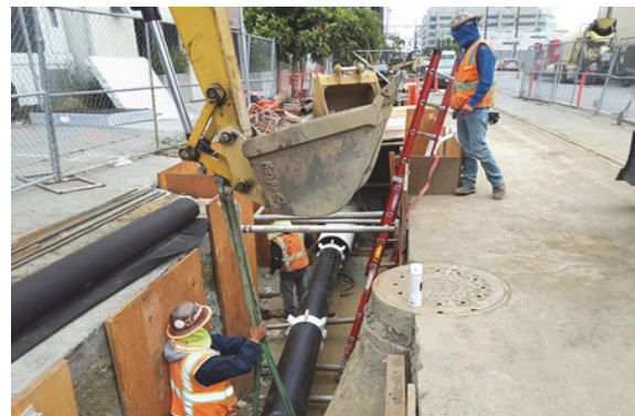
Insertion of the HDPE Force Main
