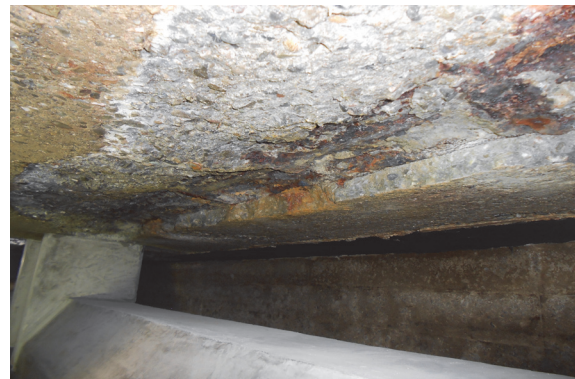
Completed weir repair and corrosion in the ceiling of Sansome CSD
