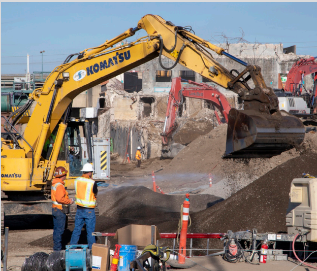
Southeast Wastewater Treatment Plant: Headworks project demolition.
