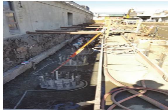
Seismic Piles on the North of SEP 042
