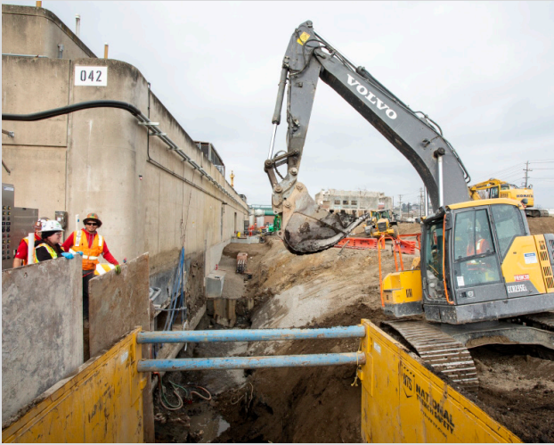
Southeast Wastewater Treatment Plant: Headworks project Excavation.
