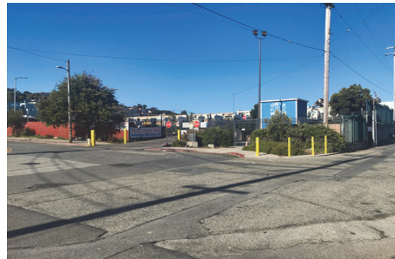
KM MTBM Receiving Area
