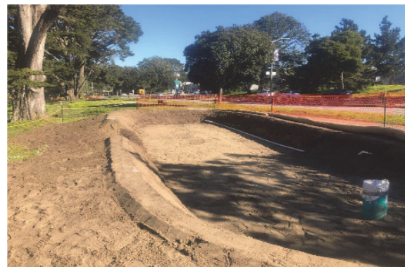
Rain garden excavation between Irving and Judah Streets
