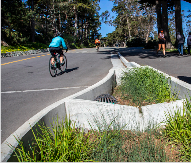
Baker Beach Green Streets: Rain gardens at El Camino Del Mar between Legion of Honor Drive to 32nd Avenue.
