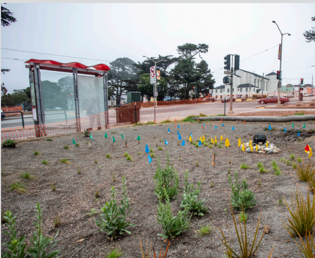
Sunset Boulevard Greenway: View of planter at 37th Avenue and Judah Street. Flags represent the variety of plants that will be planted in the rain garden.
