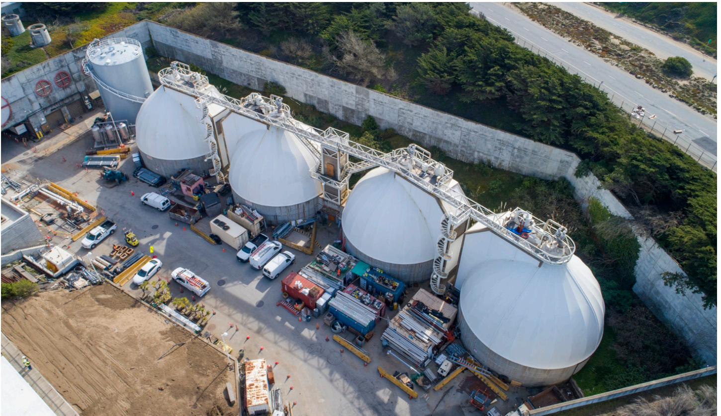
Westside Enhanced Water Recycling Project: Oceanside Treatment Plant (OSP), aerial drone view of digesters.
