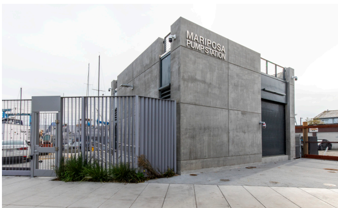
Mariposa Pump Station Improvements Project: Exterior of pump station.
