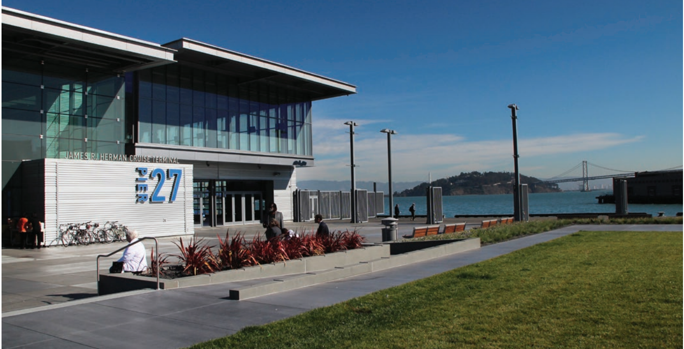
The James R. Herman Cruise Terminal at Pier 27 (image courtesy of San Francisco Public Works)
