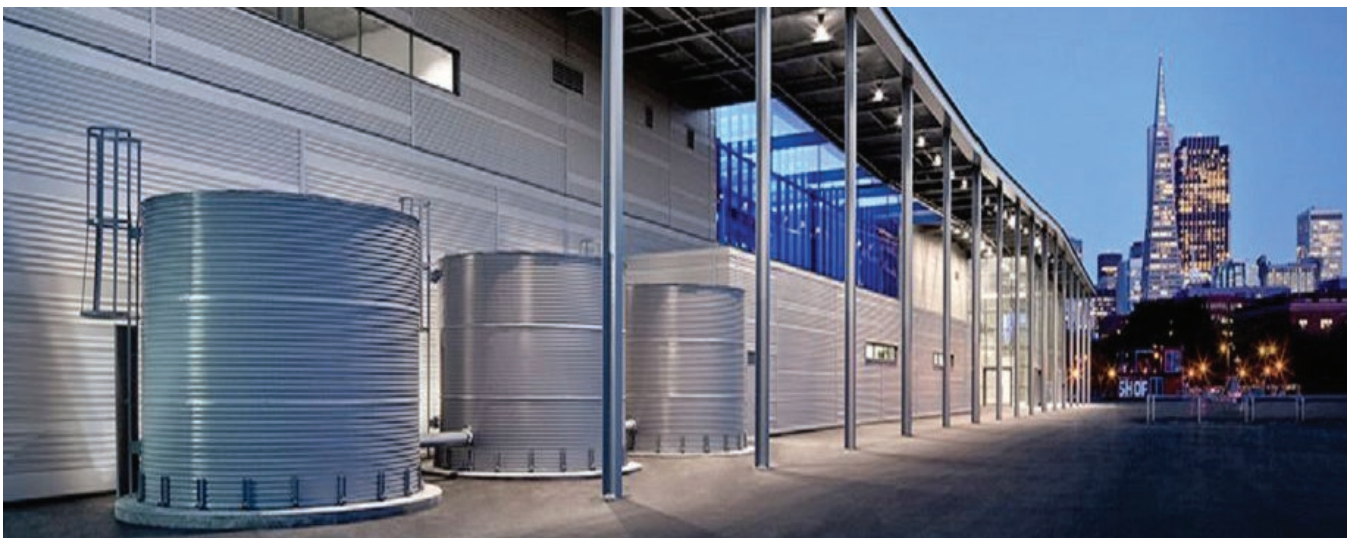
The rainwater cisterns at Pier 27 (image courtesy of San Francisco Public Works)
