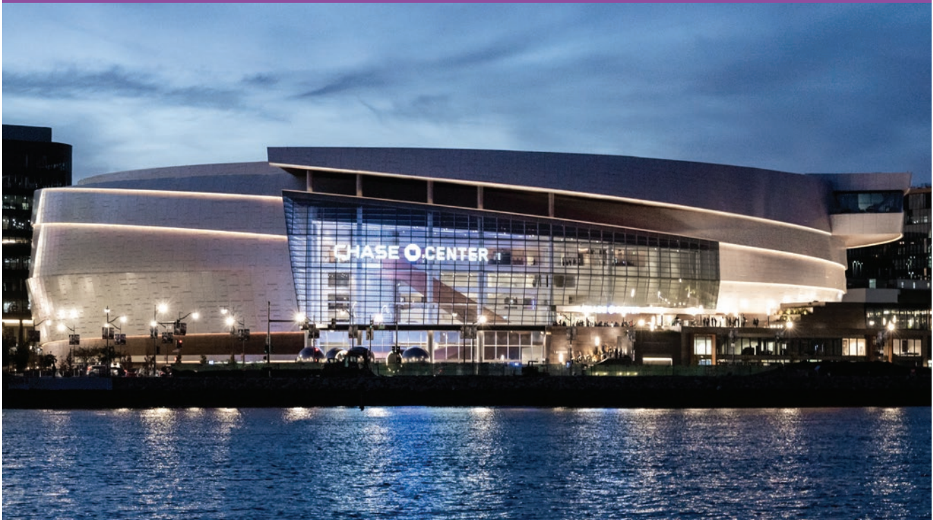
Chase Center arena (image courtesy of Chase Center)
