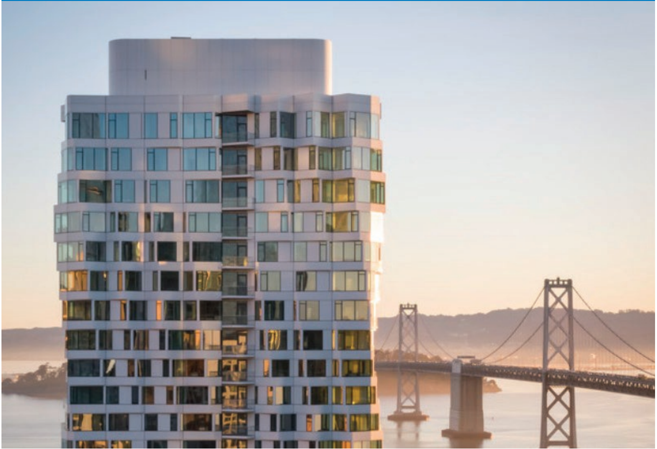
MIRA tower (image courtesy of Aquacell by PHOENIX)
