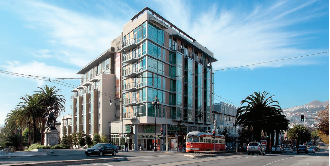
38 Dolores Street (image courtesy of BAR Architects)
