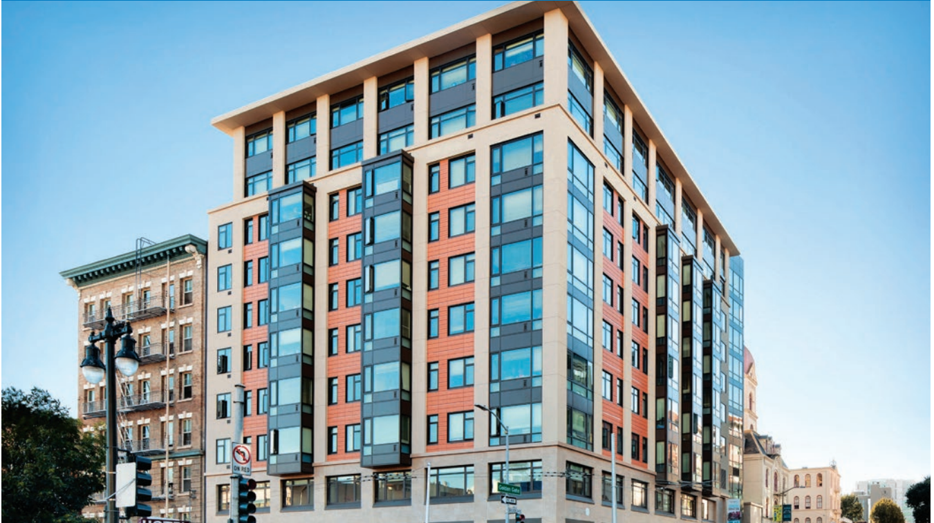
The Vera Haile Housing and St Anthony's Foundation Dining Room and Social Work Center (image courtesy of David Wakely Photography)
