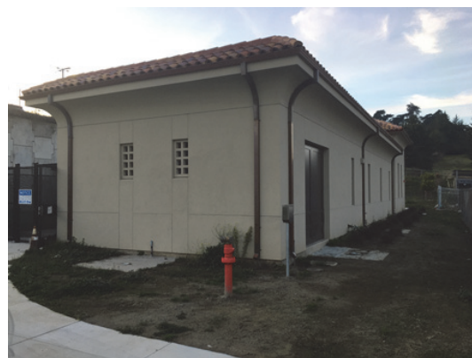
Serramonte Boulevard Well & Treatment Facility in Colma, CA
