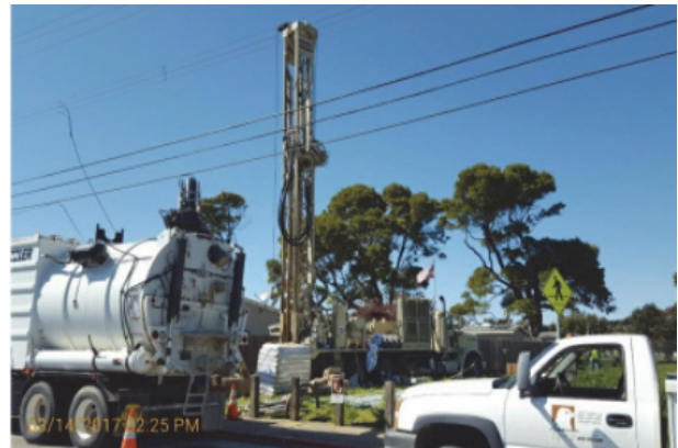
Deep Anode Installation – Corrosion Phase 1
