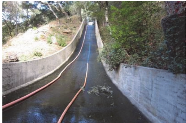
Spillway cleaning and mapping for condition assessment
