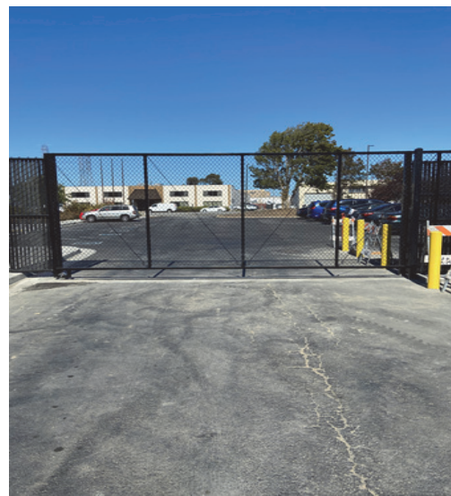
View of new entry gate at southern entrance
