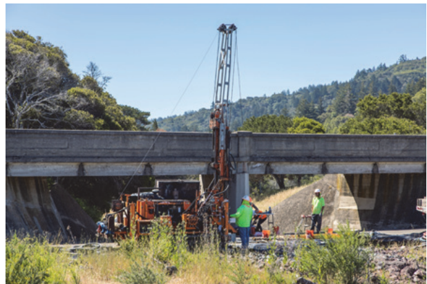
Crews performing geotechnical drilling work on dam embankment
