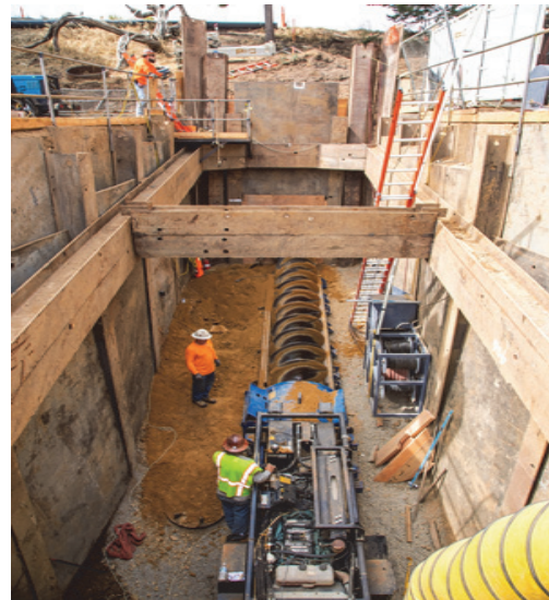
Installation of 24-inch diameter ERDIP reservoir inlet pipe.
