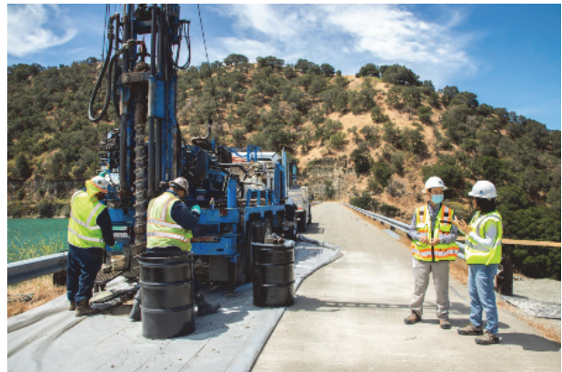
Crews performing geotechnical drilling work on dam crest during DSOD site visit
