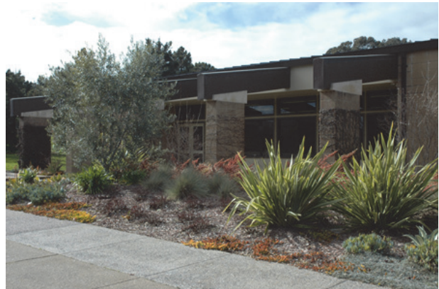
Existing Administration Building
