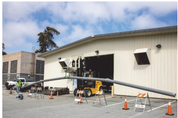
Earthquake Resistant Ductile Iron Pipe with flexible joints (demonstrated) used for this project
