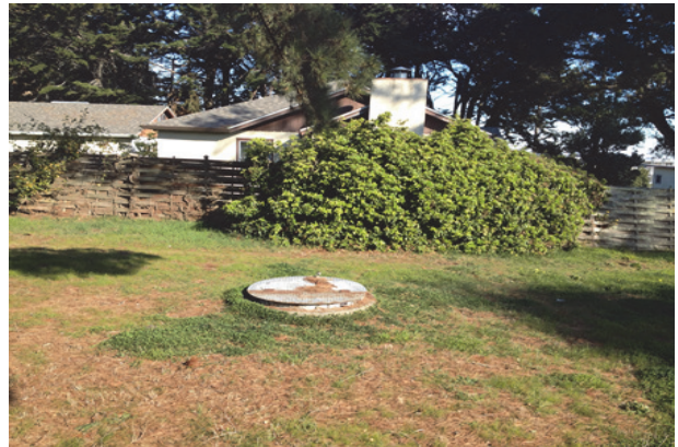
Typical Appurtenance to be Upgraded
