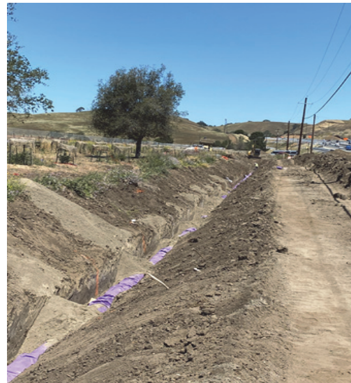
Installation of 12" Town of Sunol Raw Water Pipeline North of Hwy 680
