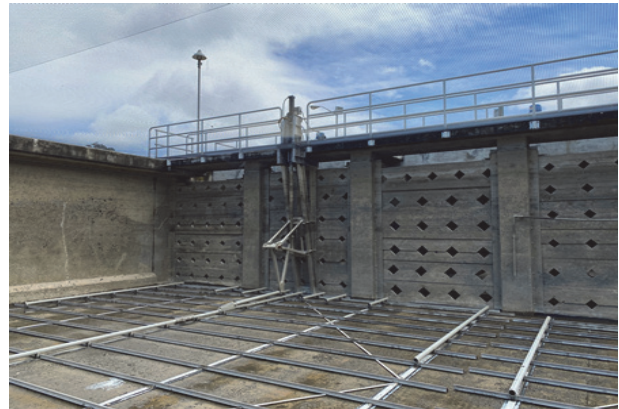
Inspection of Sedimentation Basin 1
