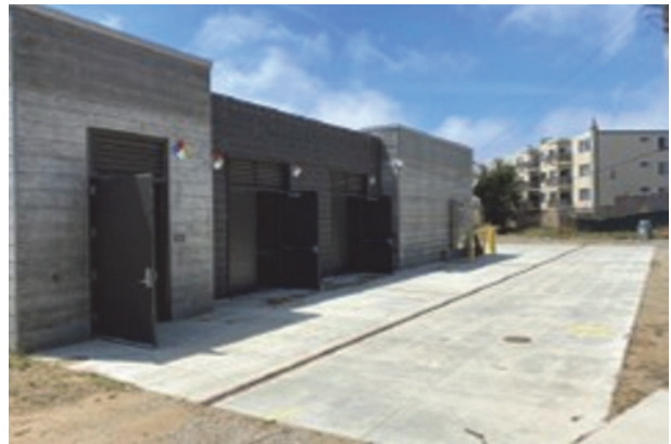
Well Station Building
