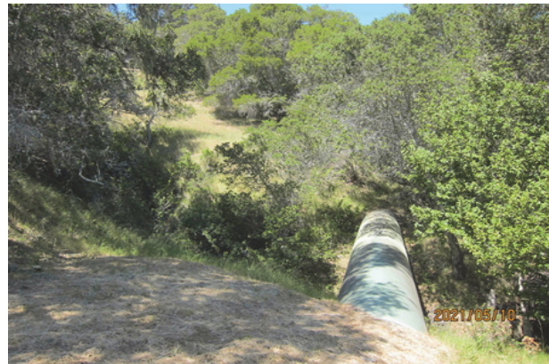
CSPL2 Gully Crossing
