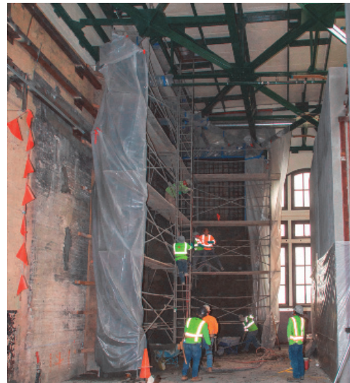
Roof installation of Pump Station No. 2
