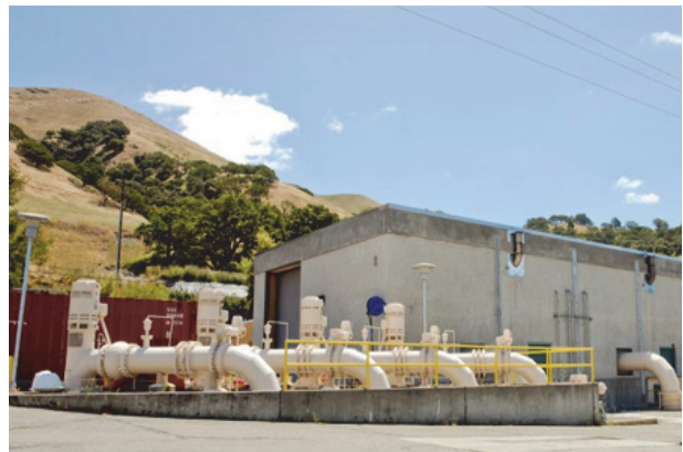
San Antonio Pump Station building looking southeast
