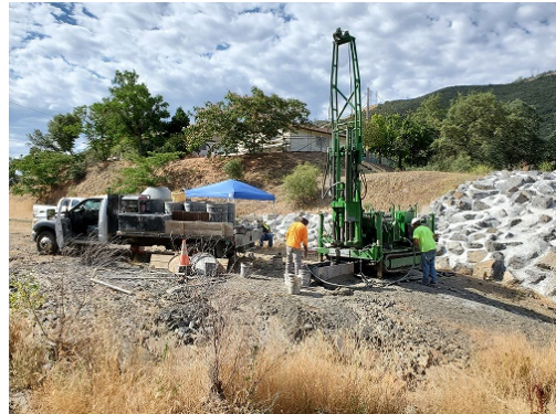
Moccasin Geotechnical Drilling
