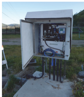
Sunshade installed for the water quality equipment
