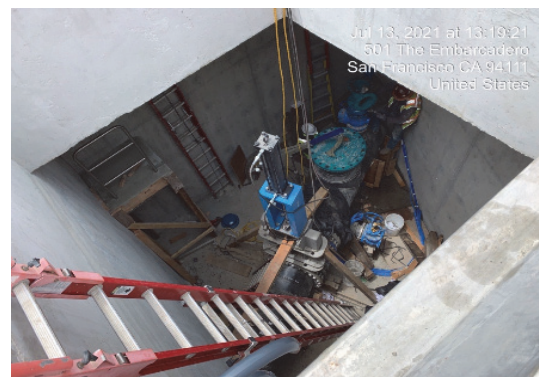
New Force Main and Appurtenances Inside New Valve Vault
