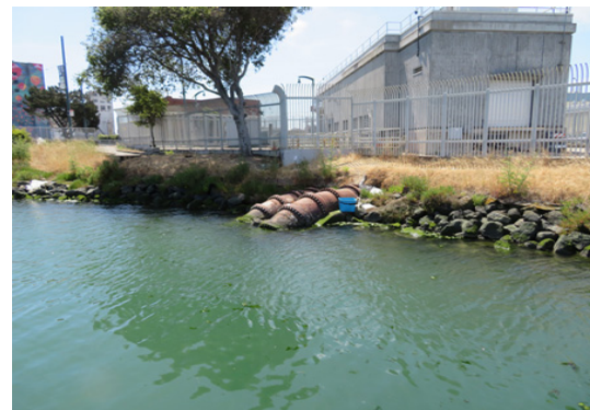
Current pipeline crossing at Islais Creek
