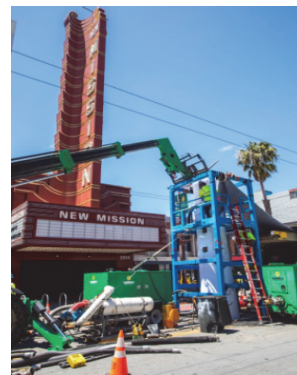
Performed Cured-In-Placed lining process along Mission Street
