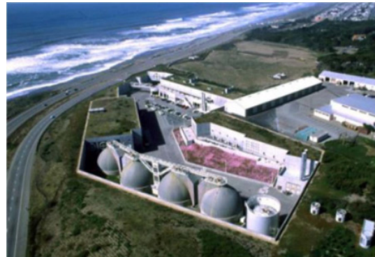
OSP Site Aerial Photo
