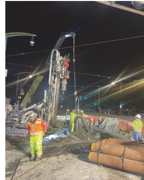
Driving Micropiles for Offset Manhole
