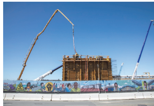
Grit Handling Building wall construction (Evans Ave view)
