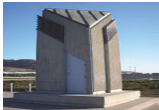
Sunnydale Pump Station
