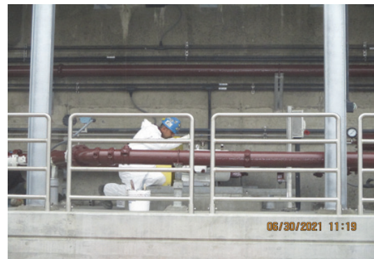
Scum System Installation
