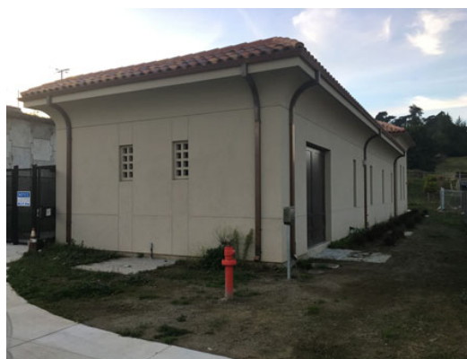
View of Poncetta Drive Well & Treatment Facility in Daly City (formerly named Lake Merced Golf Club Well Station)
