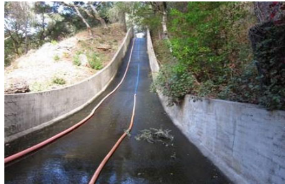
Spillway cleaning and mapping for condition assessment
