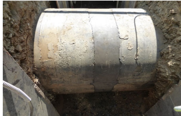
Pipeline excavated for corrosion investigation
