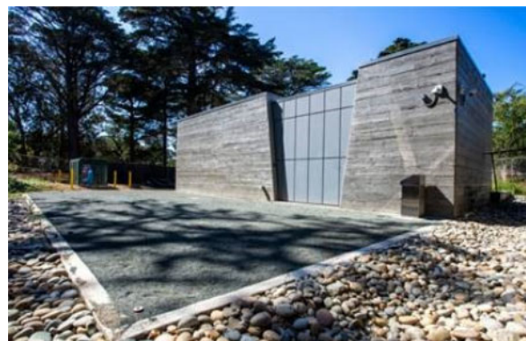
North Lake Well Station
