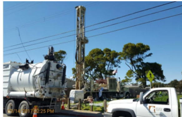
Deep Anode Installation – Corrosion Phase 1
