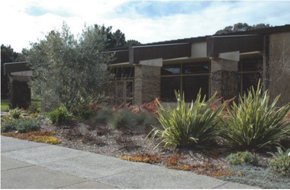
Existing Administration Building
