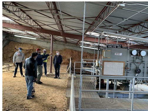
Site visit inside West Portal Valve House
