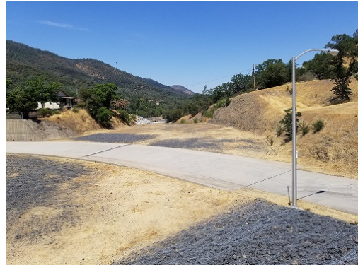
Moccasin Dam Existing Auxiliary Spillway
