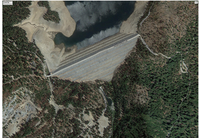
Cherry Valley Dam and Spillway
