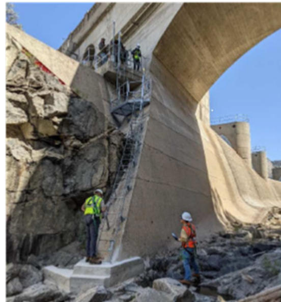
Exterior Ladder and Fall Protection to Spillway Invert
