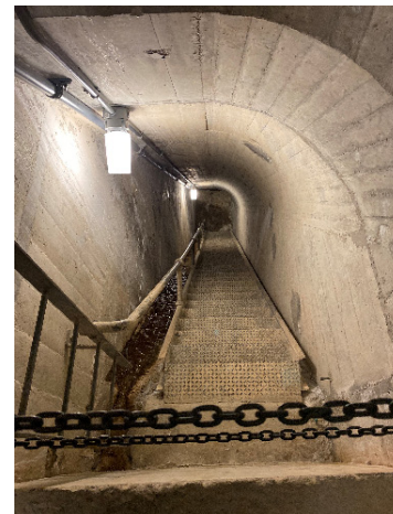
Inclined Stairway OSH Dam
