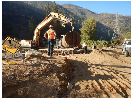
Oil Water separator tank removal at Kirkwood Powerhouse
