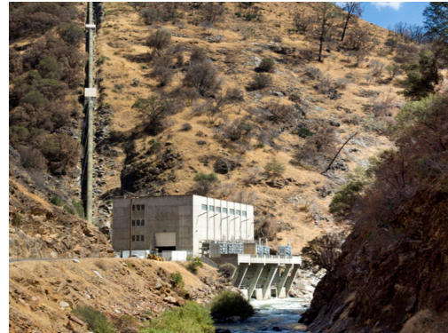
Generator Shaft at Moccasin Powerhouse
