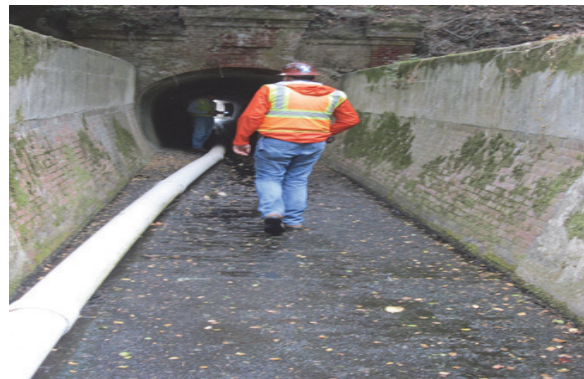
Pilarcitos spillway inspection
