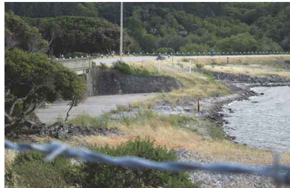
San Andreas Dam and Spillway
