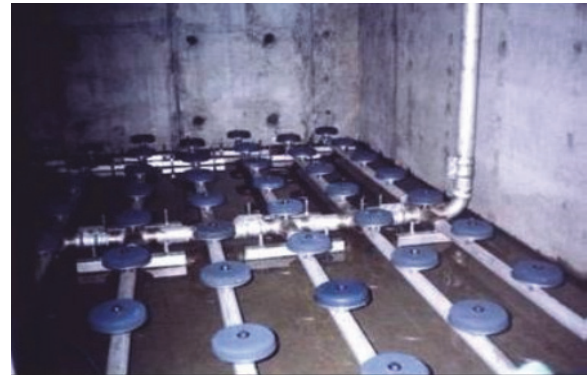
Example of Fine Bubble Diffusion Ozone Application System
