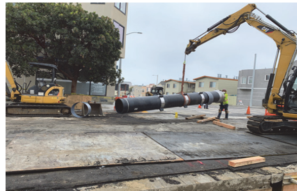
WD-2766 Taraval Casings under Tracks
