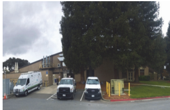
Existing Millbrae Administration Building
