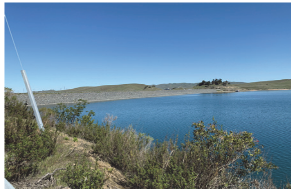
Upstream Face of Turner Dam and San Antonio Reservoir
