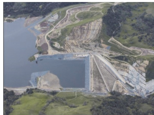
CDRP Aerial View
