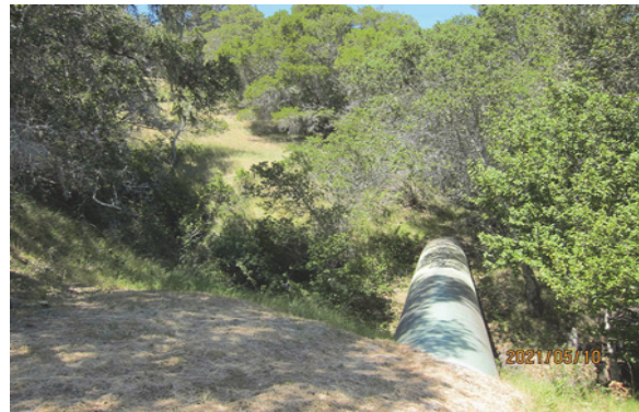
CSPL2 Gully Crossing with Limited Vehicle Access
