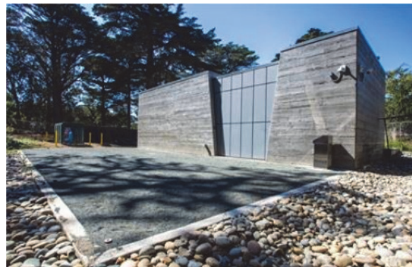
North Lake Well Station
