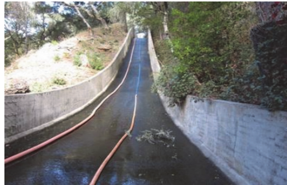
Spillway cleaning and mapping for condition assessment
