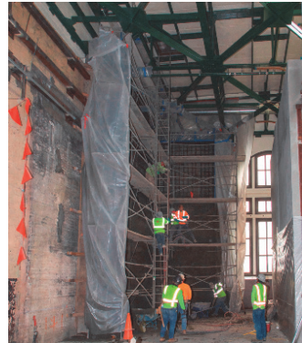
Roof installation of Pump Station No. 2
