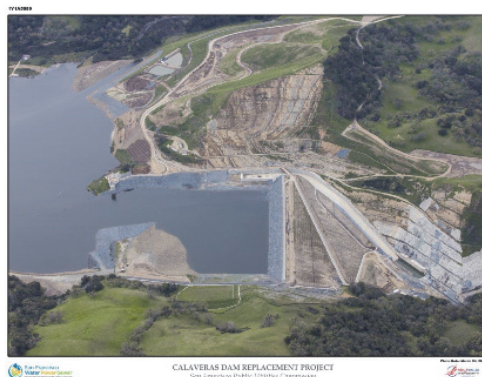
CDRP Aerial View
