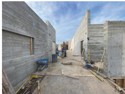
Architectural Concrete Walls at Building Entrance
