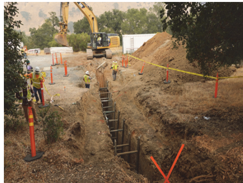
Geotech fault trenching across the site
