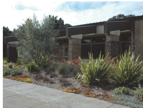
Existing Administration Building
