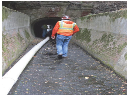
Pilarcitos spillway inspection
