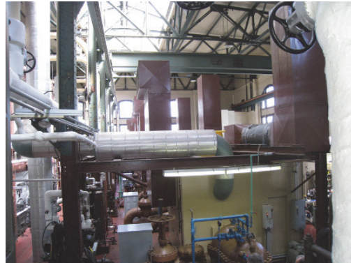
Interior view of PS2 showing a pump, valves, engine sound enclosure and exhaust, and building structural members
