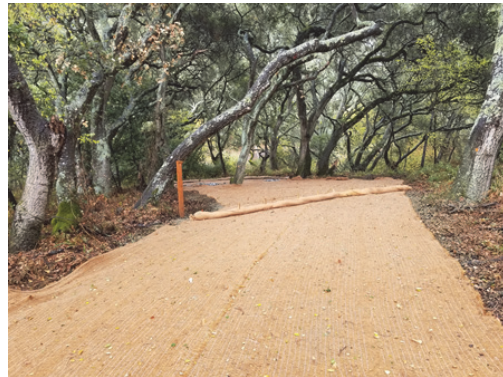
Site restoration work at Segment 1
