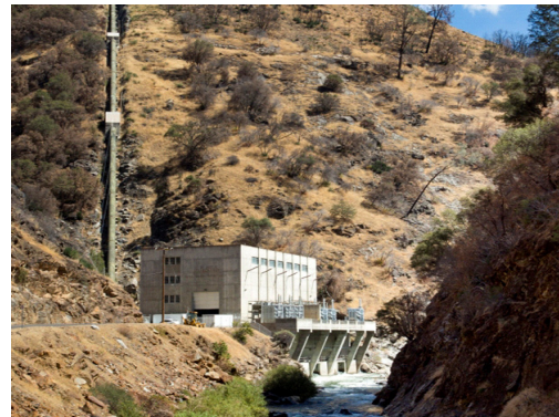
Generator Shaft at Moccasin Powerhouse
