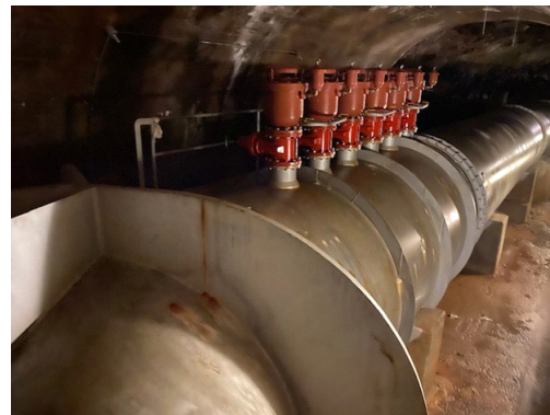
Diversion Pipe at O' Shaughnessy Dam
