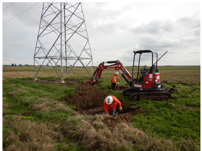
Potholing Existing San Joaquin Pipelines 1, 2, and 3 at Tower 518S
