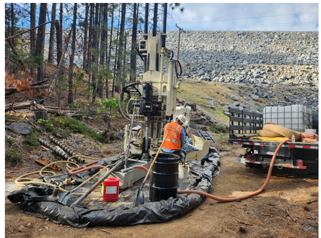
Cherry Valley Dam Spillway Geotechnical Exploration
