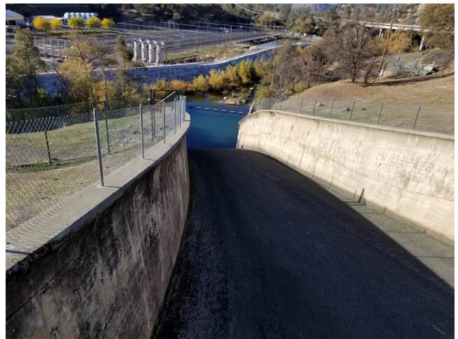
Moccasin Dam Spillway Chute
