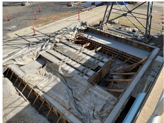
MPH HH-1003R GSU2 Foundation
