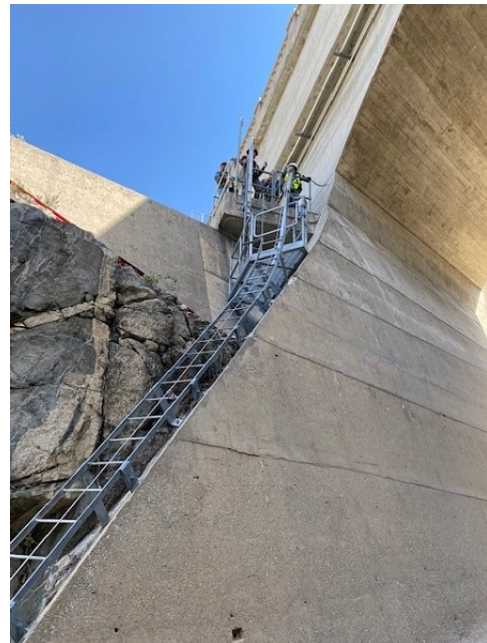
Spillway Access Ladder
