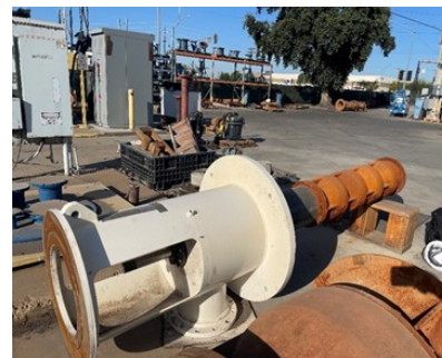
Inspection of the Vertical Pump
