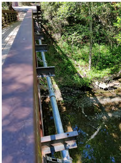
New Water Line Installed on Headquarters Bridge
