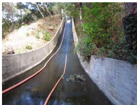
Spillway cleaning and mapping for condition assessment
