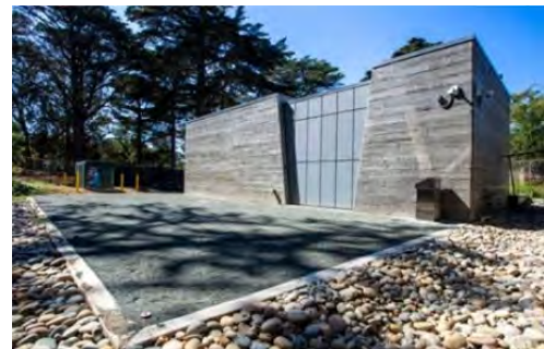
North Lake Well Station
