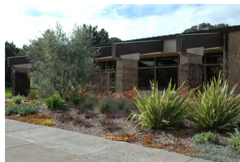
Existing Administration Building
