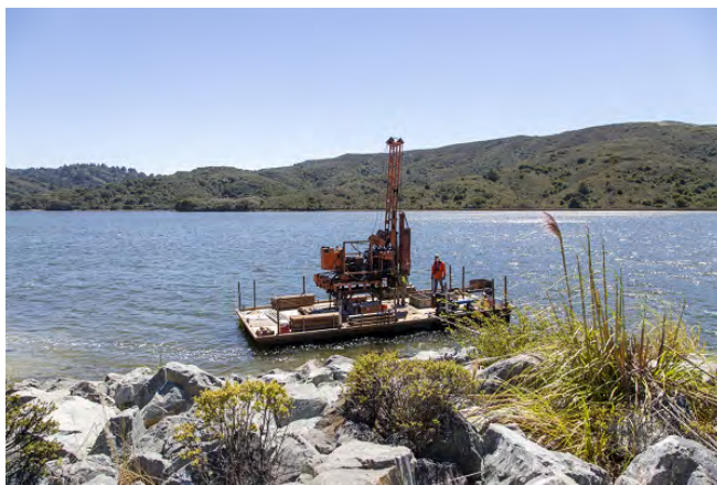
Barge Launch for Geotechnical Drilling into Lake
