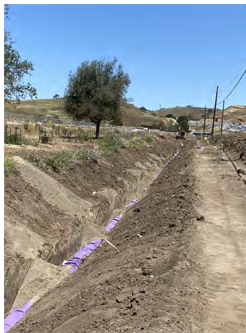
Installation of pipeline by Highway 680
