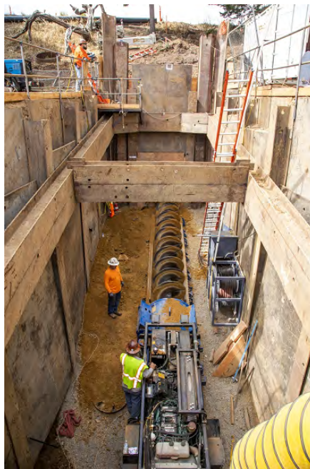
Installation of 24-inch diameter ERDIP reservoir inlet pipe
