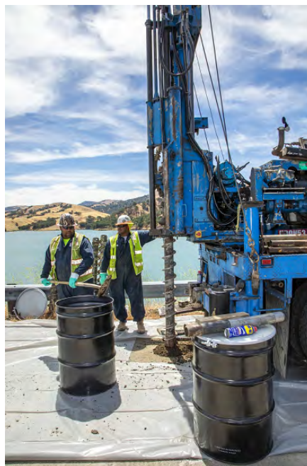
Geotechnical Drilling Core of Dam
