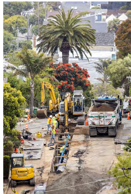
Prospect Avenue Water Main Replacement
