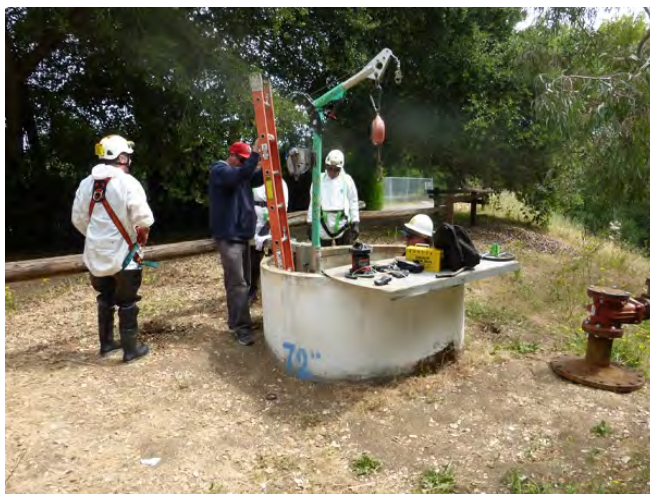
Example of Equipment for Worker Safe Pipeline Entry
