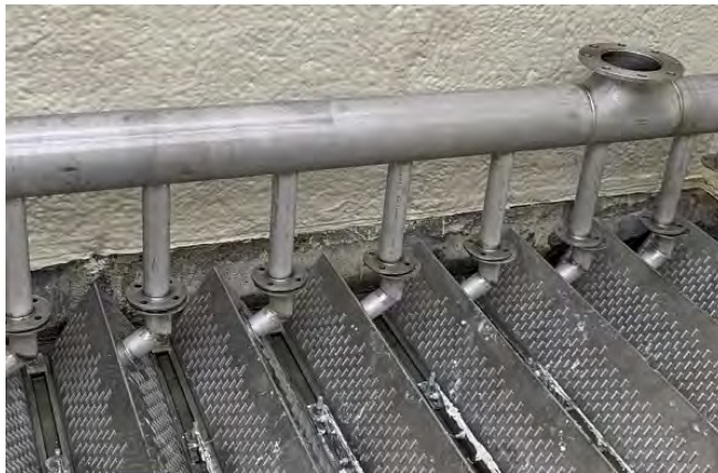
Proposed Stainless Steel Underdrains and Air Piping
