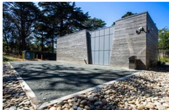
North Lake Well Station
