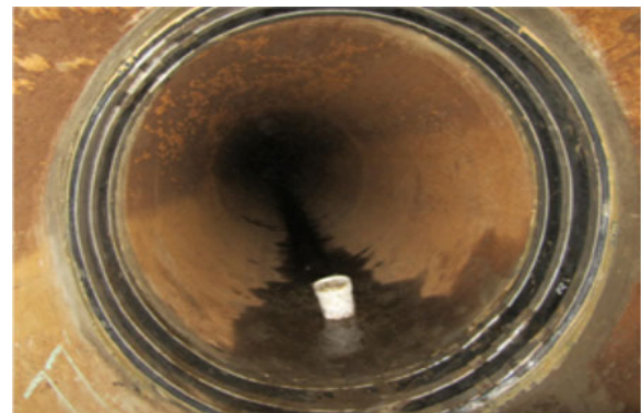
Typical Pipeline Repair with WEKO Seals
