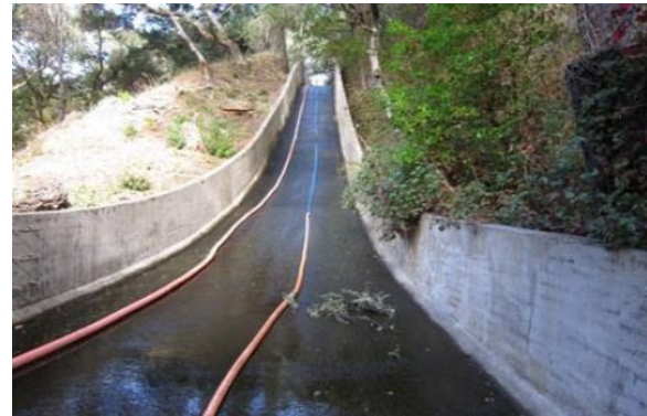
Spillway cleaning and mapping for condition assessment
