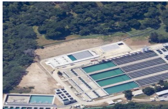
Sunol Valley Water Treatment Plant Basins 1-5
