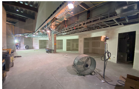
Drywall and Framing of the History Alcove and Interpretative Display Areas
