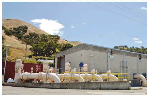
San Antonio Pump Station building looking southeast
