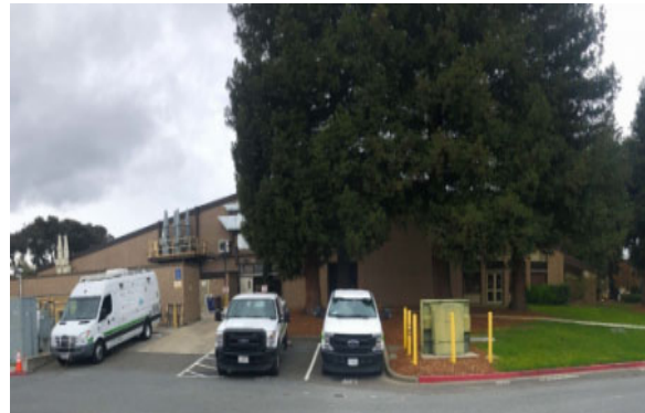
Existing Millbrae Administration Building
