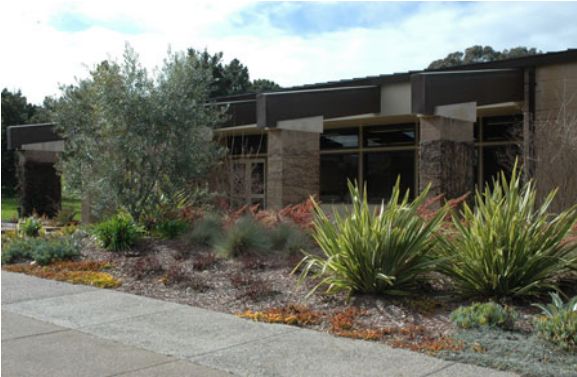
Existing Administration Building
