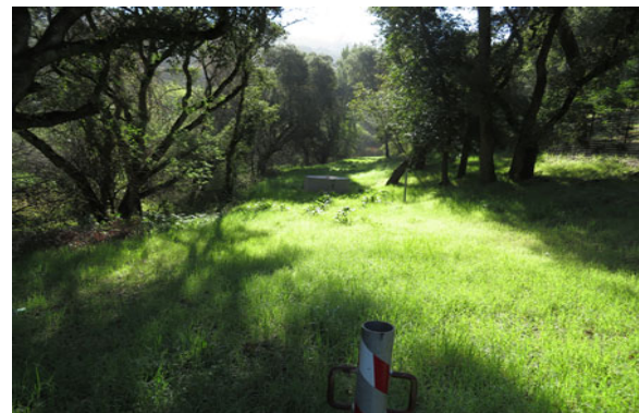
Portion of CSPL2 that will be re-lined
