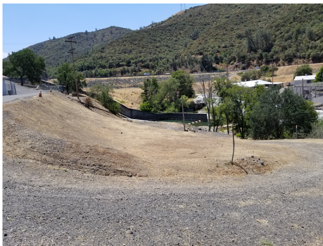
Moccasin Dam and Spillway
