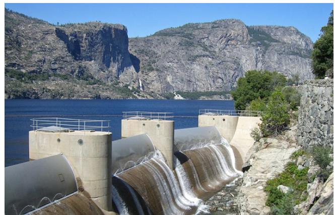
O'Shaughnessy Dam Spillway and Drum Gates
