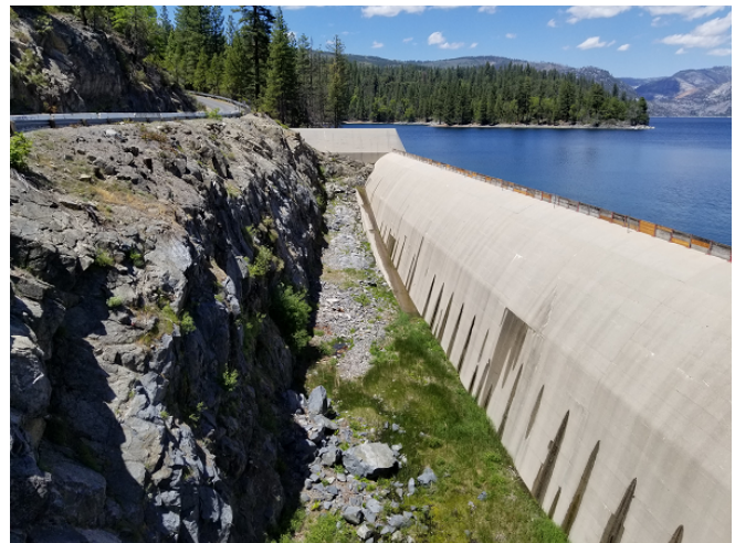
Cherry Valley Dam Spillway
