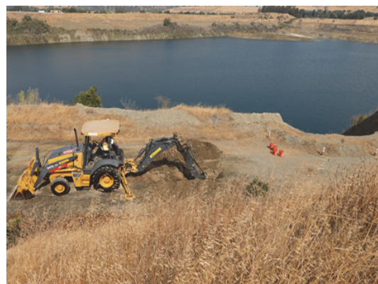
Geotech Investigating Trenching at Pond F2
