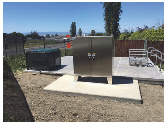
Ventilation and Sump Pump Project
