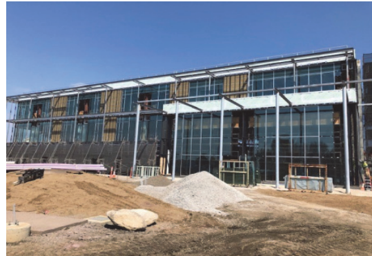
Southeast Community Center construction work in progress
