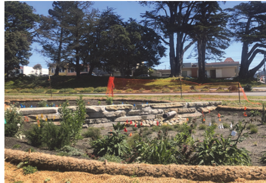
Rain garden view from east from Sunset Blvd.
