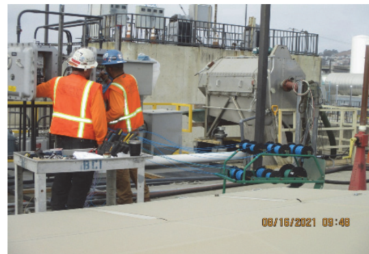
Drum Screen Wire Installation
