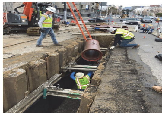
Sewer construction along Van Ness
