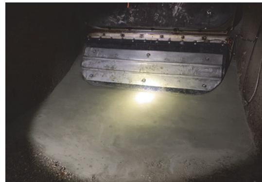
Re-installation of the Beach St. CSD backflow valve over the weir
