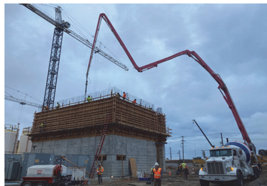
Concrete pour at new Primary Switchgear Building SEP 032
