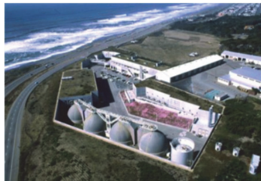
OSP Site Aerial Photo
