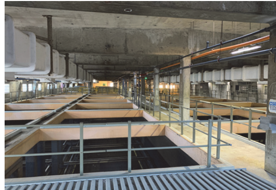
Existing SEP-041 wet-weather primary sedimentation building.
