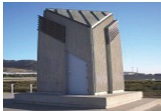
Sunnydale Pump Station
