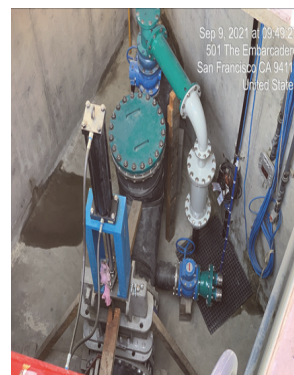
New Finished Vault and Appurtenances
