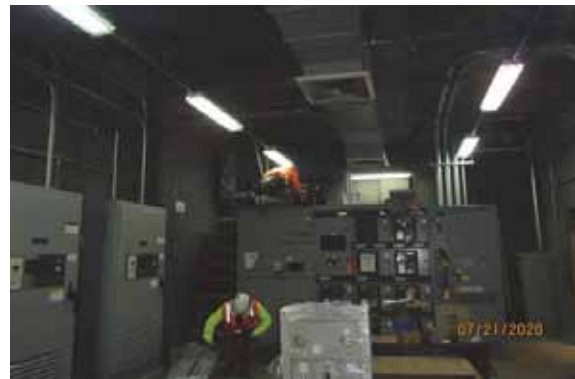
WW-651: Switchgear work during PG&E shutdown
