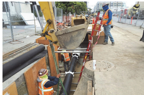
Insertion of the HDPE Force Main
