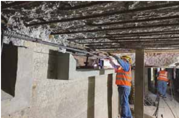
Rebar replacement on the ceiling of Sansome CSD
