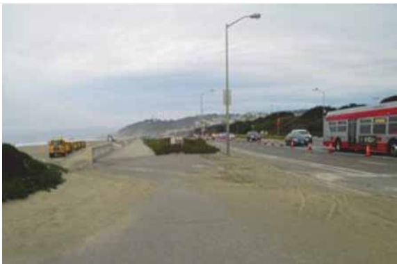
Contractor excavator and dump trucks loaded with surplus sand collected at North Ocean Beach
