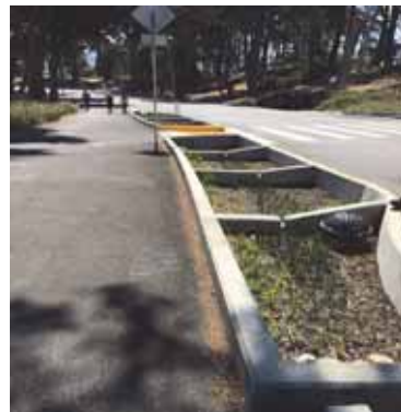
View of north side of Node 2 looking east
