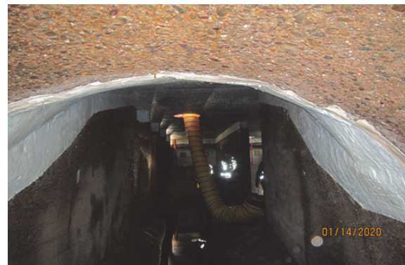
Looking into repaired 5th St. CSD discharge pipe
