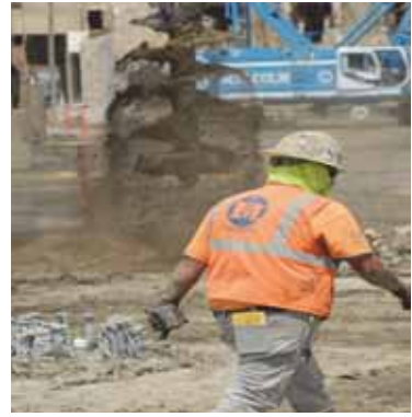
Scope III - Earthwork/Drilled Piers
