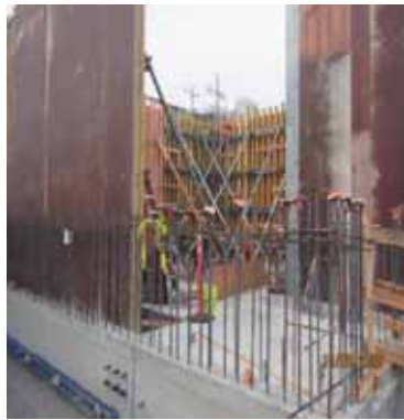
WW-667: Setting formwork for the 1st level
