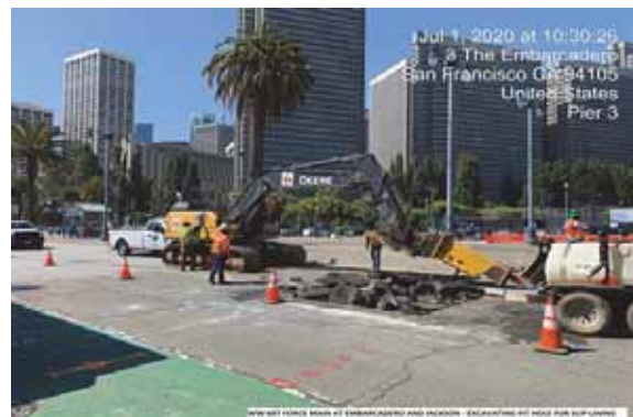
WW-687: Excavating Pit Hole for Slip-Lining
