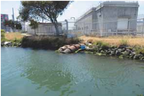
Current pipeline crossing at Islais Creek
