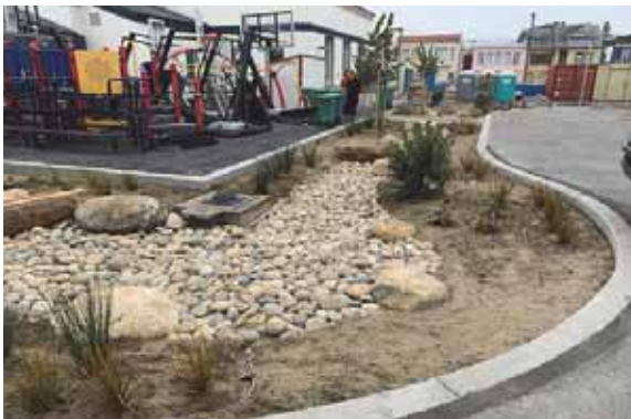
View of Lafayette Elementary School Green Infrastructure Construction
