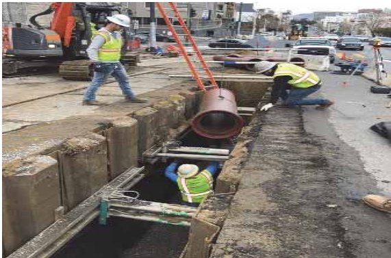
Sewer construction along Van Ness
