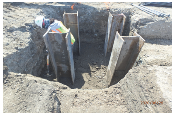
Pile driving completed
