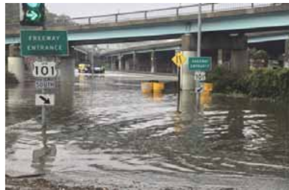
Flooding at the I-280/Hwy 101 interchange at Lower Alemany area, during the rainfall of February 13, 2019
