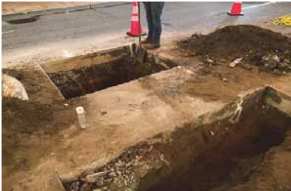
WW-696: Potholing along 3rd Street
